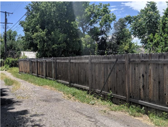
View of fence along alleyway (east property line)
