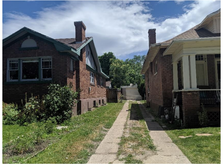
Adjacent home and driveway to the south on Lake Street (right)
