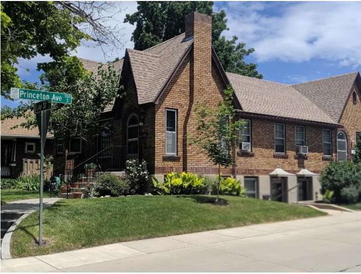
Adjacent home to the north on Lake Street (right)
