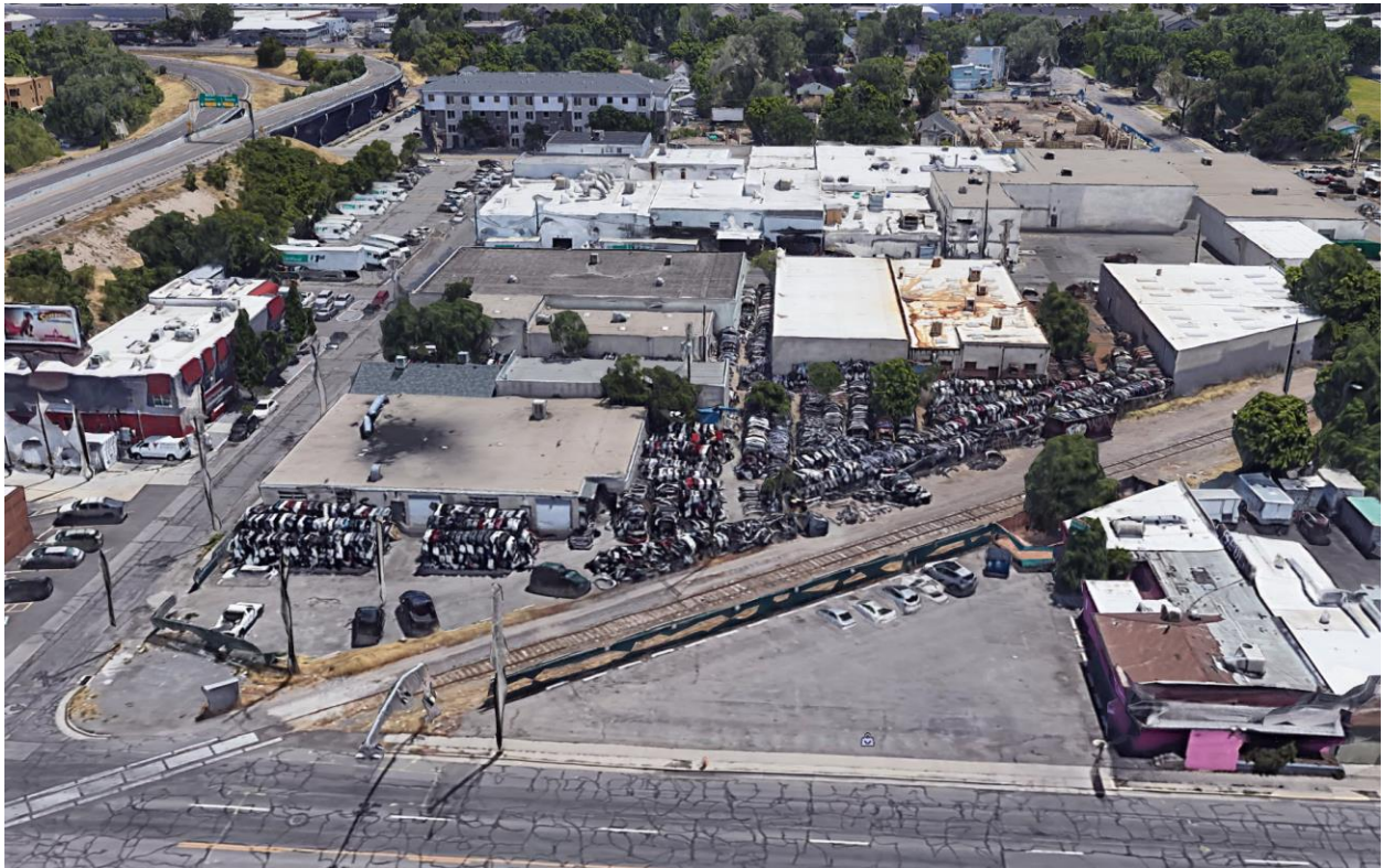
View from above looking east of 300 W.
