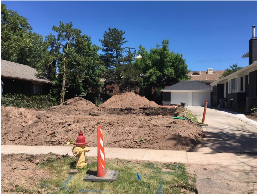
Subject property looking north – garage is shared between 815 and 819 Emerson
