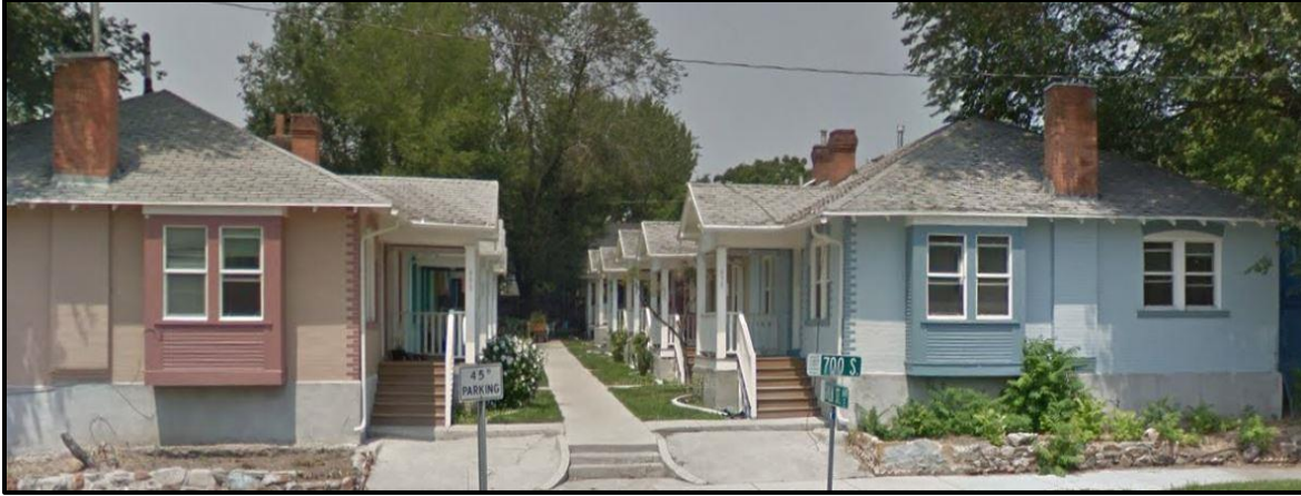
661 S. Green St. – 10 units on 27,234 sq. ft. = 2,723 sq. ft. per unit Current Allowance 9 units (separate structures on single lot also not permitted)
