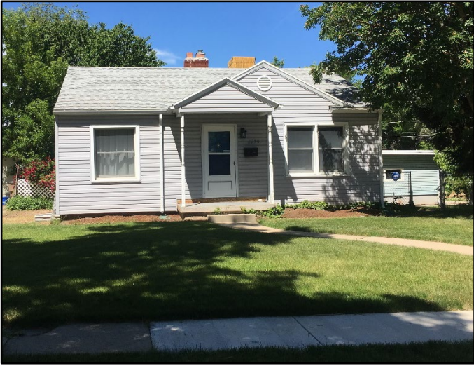
Front of existing home from 1800 East
