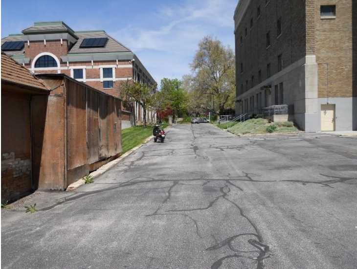
View of the driveway approach from South Temple Street looking north.
