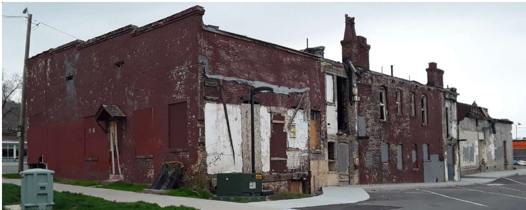
Figure 4: Existing Building, North/West Facades
