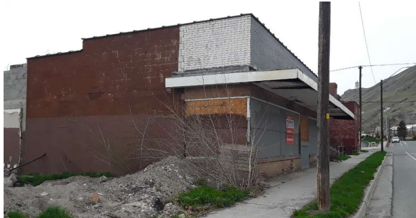
Figure 3: Existing Building, South/East Facades
