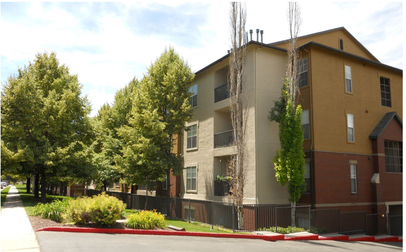
Irving Schoolhouse (looking south from the north end)
