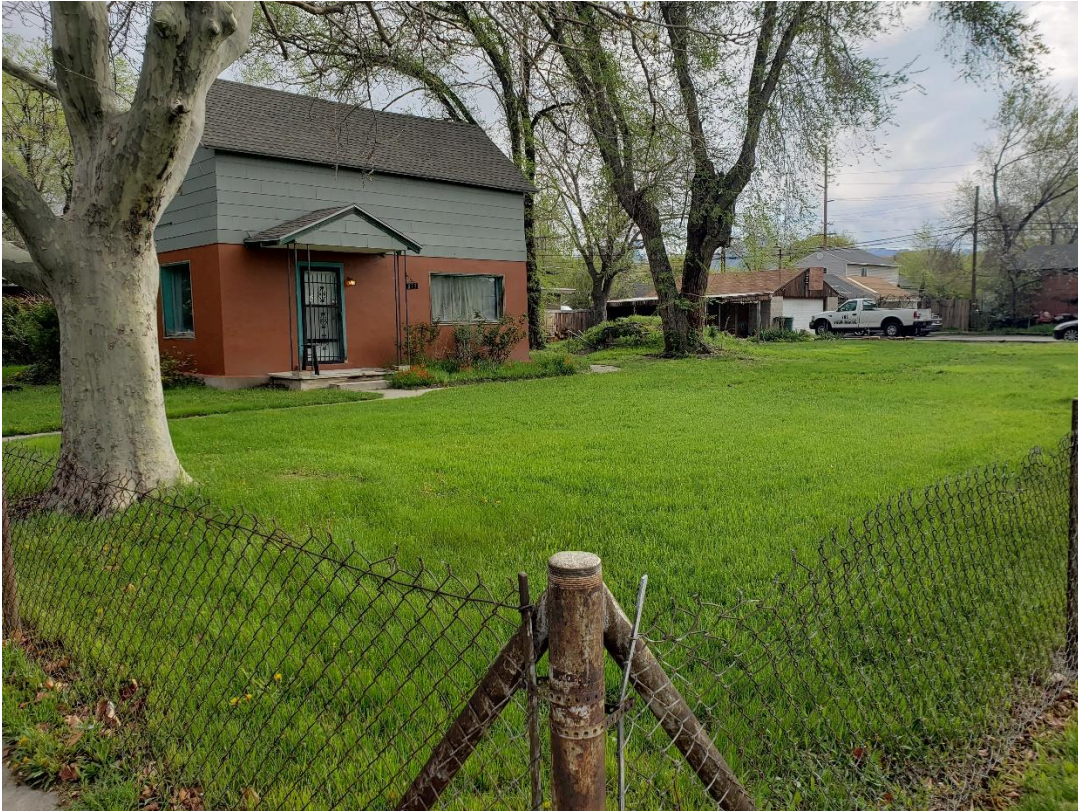
View of the current structure on the development property from the corner of 1500 West 900 South
