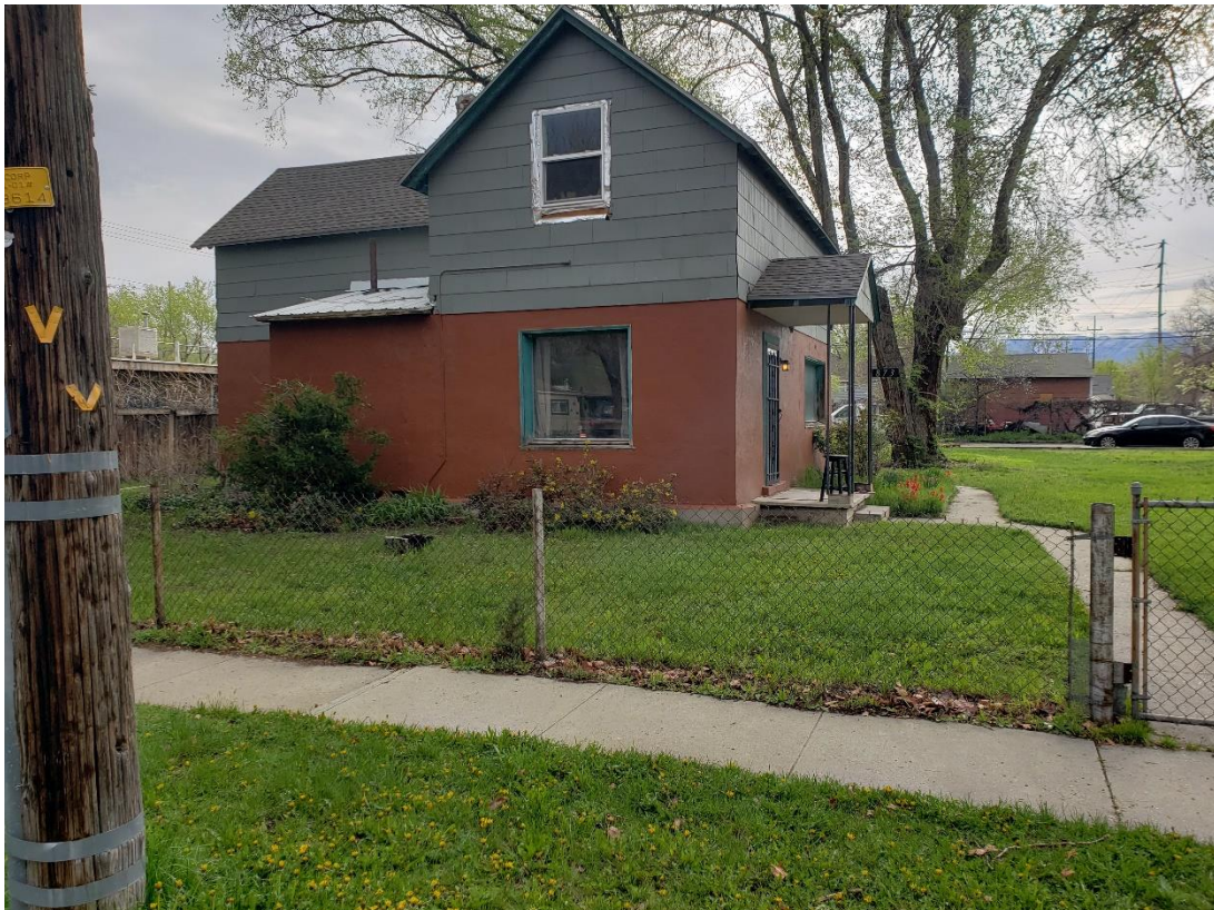
View of the home that is to remain (north side of existing lot)
