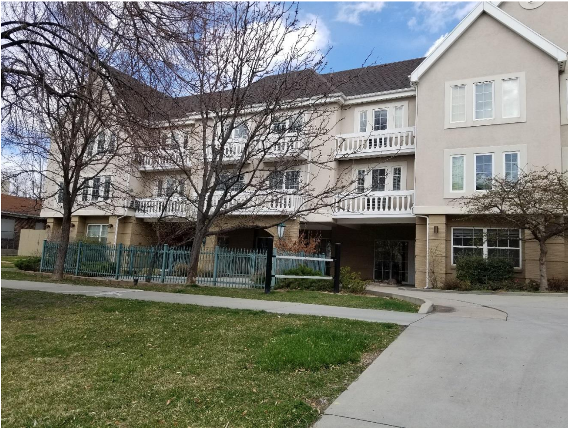
Figure 1 – Front façade of the existing building. No exterior changes are proposed.
