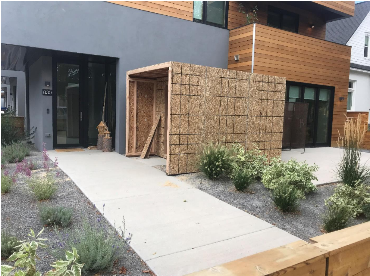
Proposed accessory structure under construction
