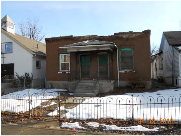
Eastward view of 833 S 200 West Street
