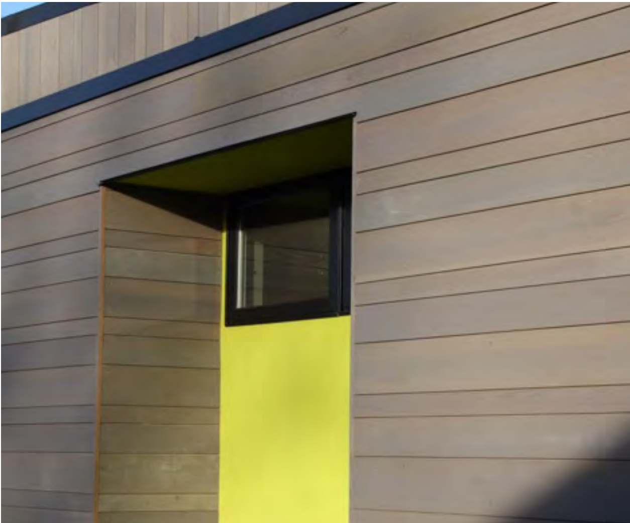
High performance windows and cedar siding
