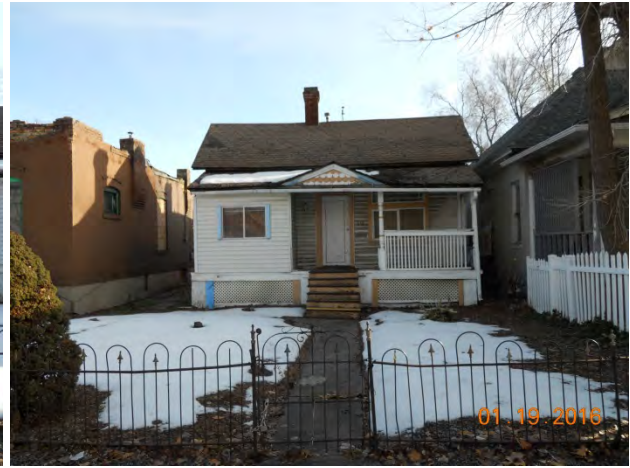
Eastward view of 839 S 200 West Street
