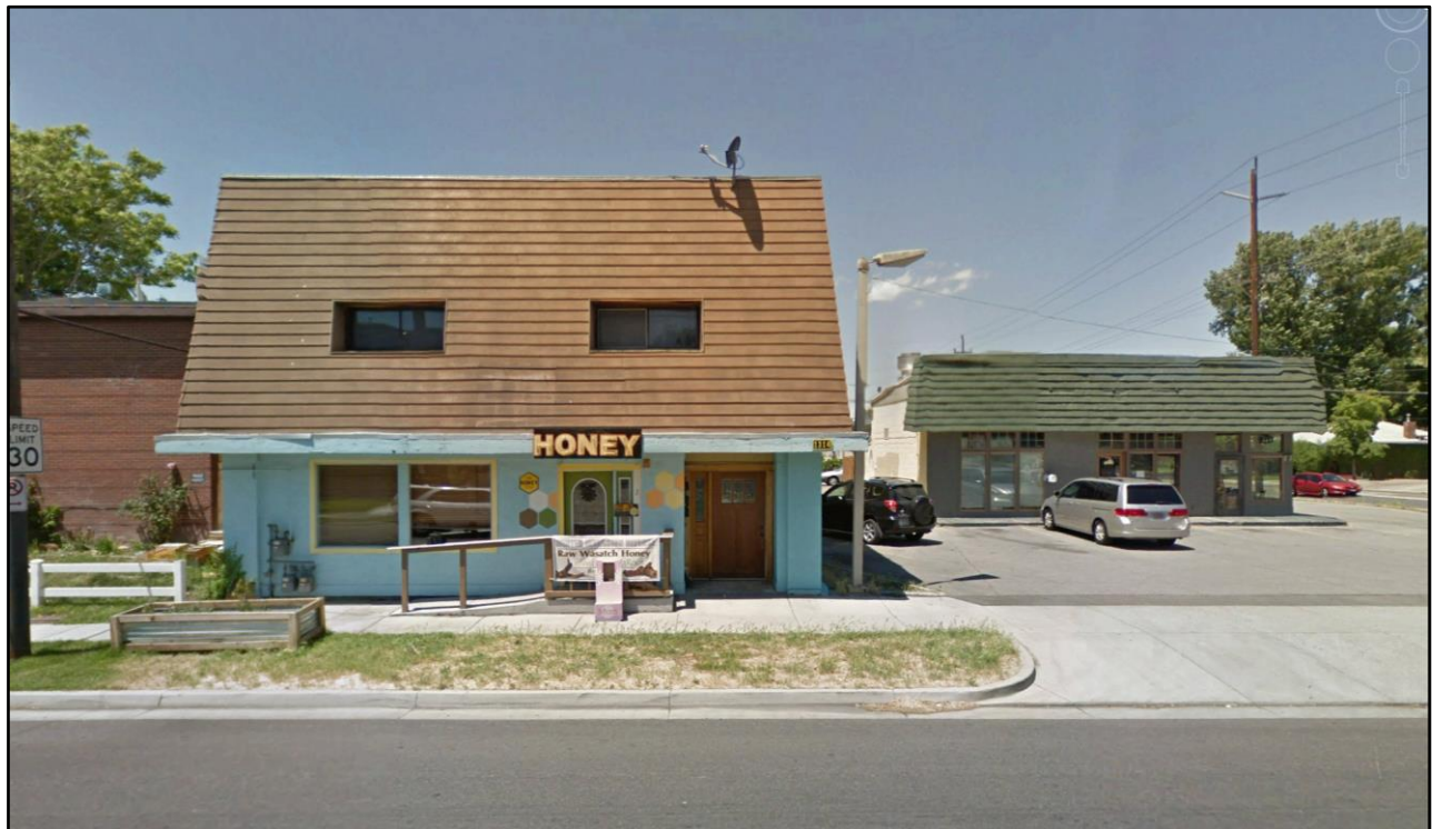
View of the South (Honey) building and the former Thai restaurant looking towards the west
