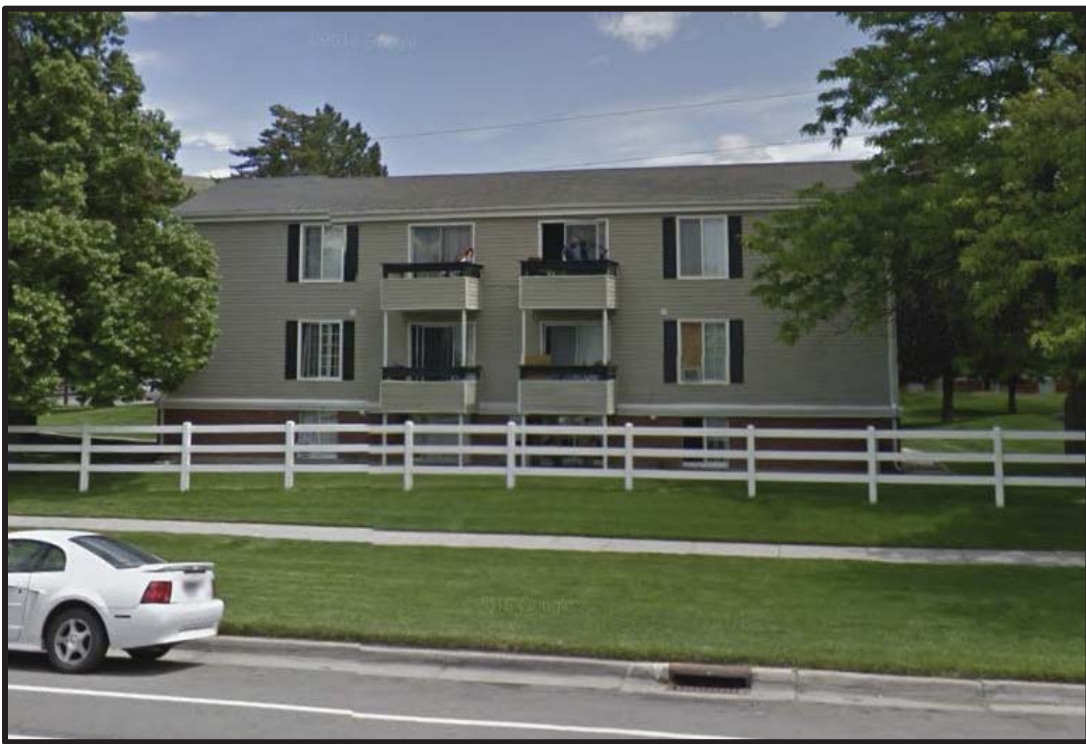
View of typical Solara apartment structure from 900 West
