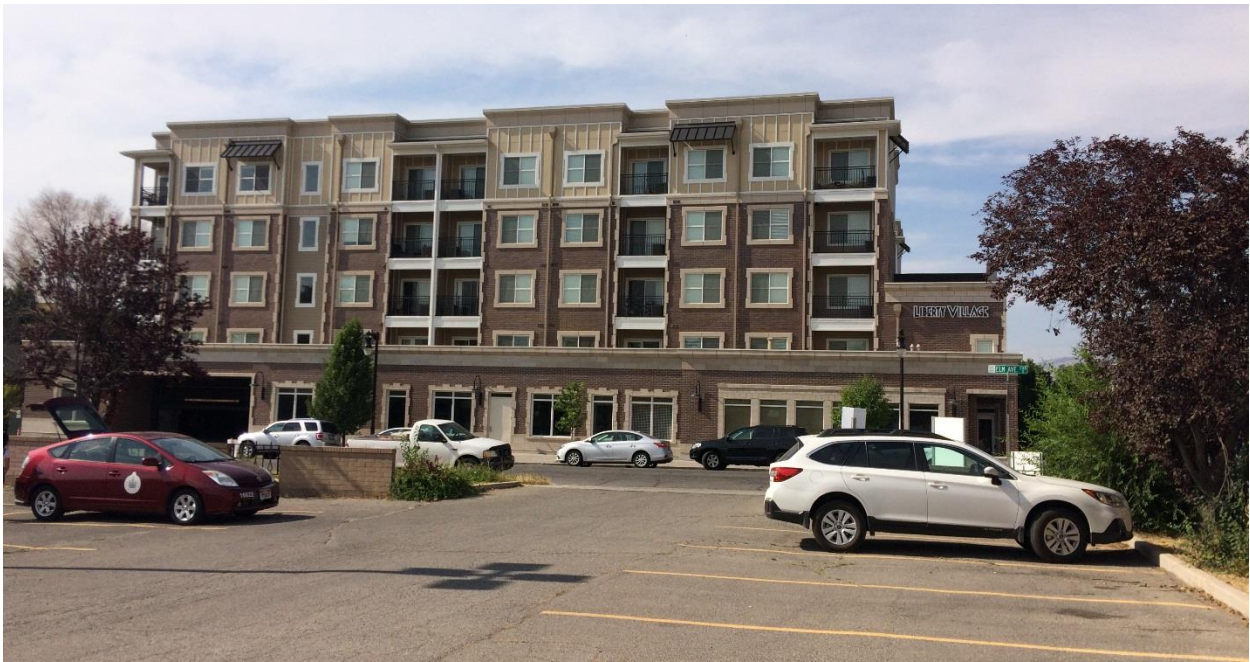
View looking north from existing site toward apartment building across the street on Elm Ave.
