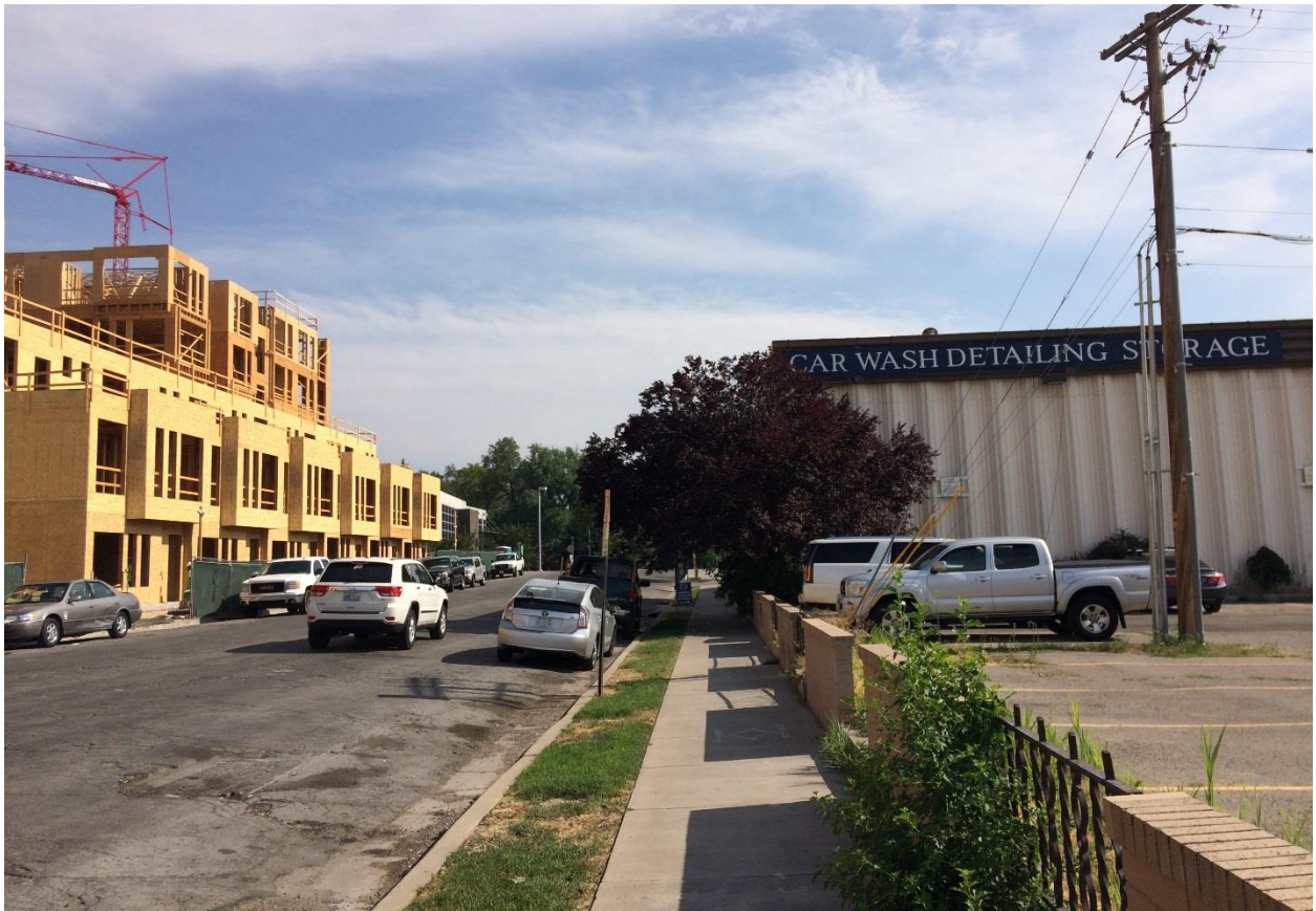
View down McClelland Street looking south, showing adjacent building (to remain) and new construction across the street to the east.
