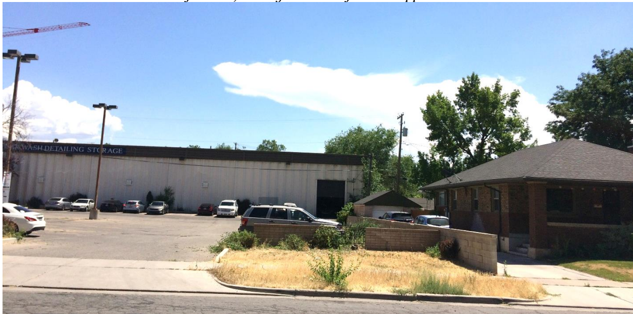
View of the west side of the property, looking south.
