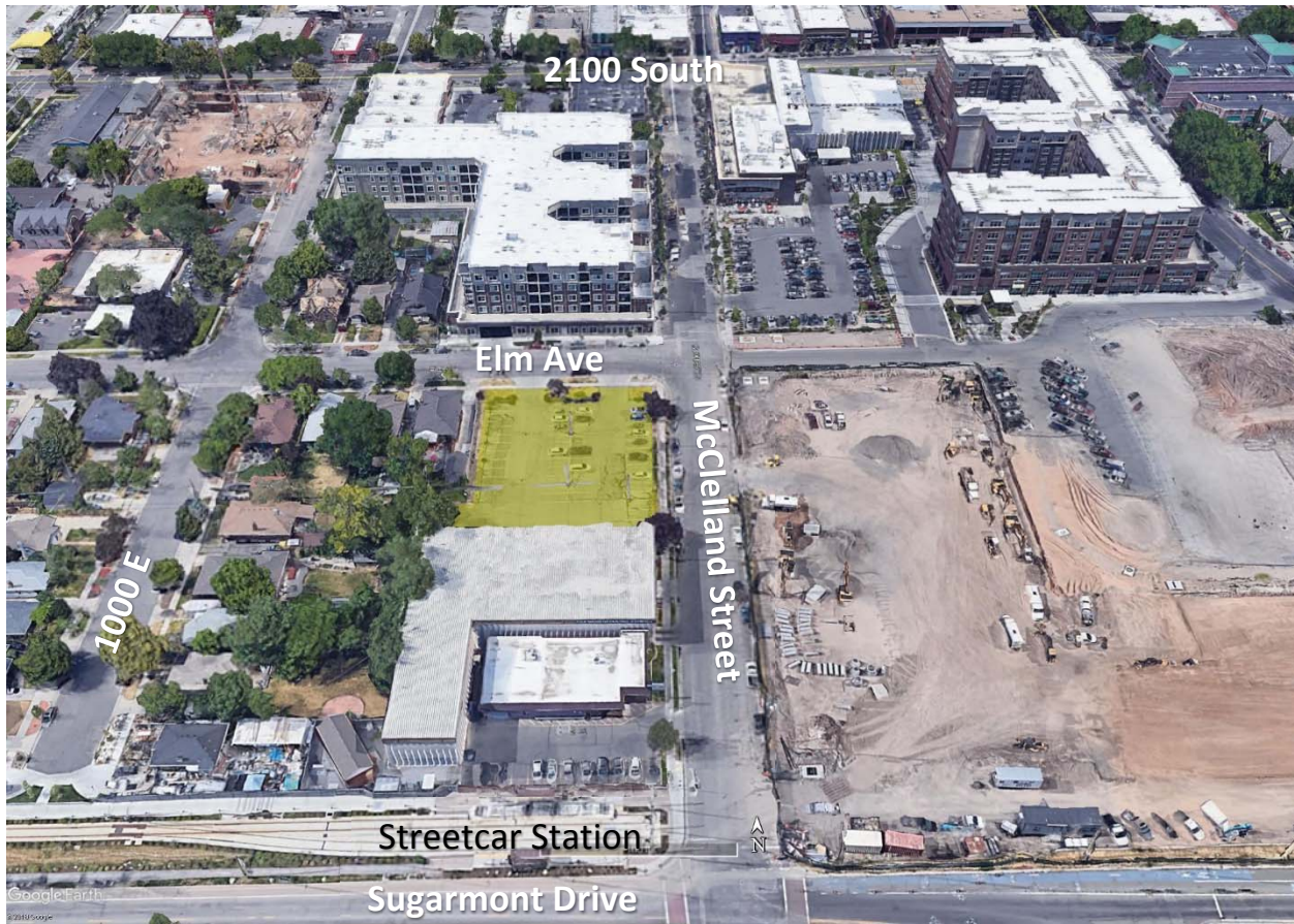
Birds-eye view of the site, looking north. Site is highlighted in yellow in the center of the aerial.
