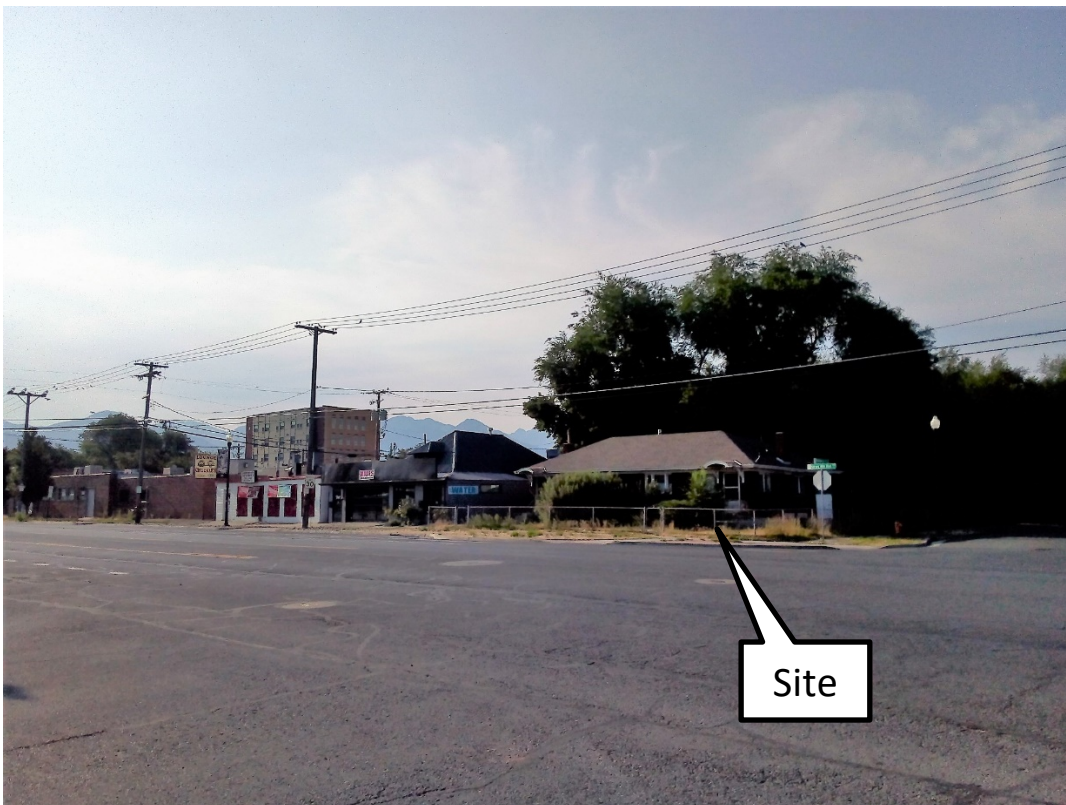
View of the subject property looking southeast across 900 South (note adjacent building heights to left of site).
