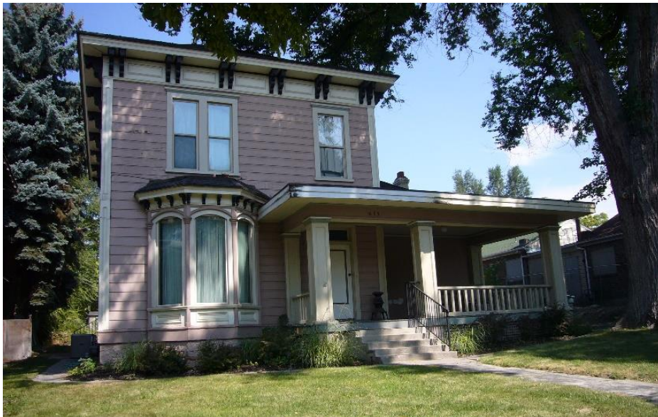
635 East 100 South (Landmark Building)
