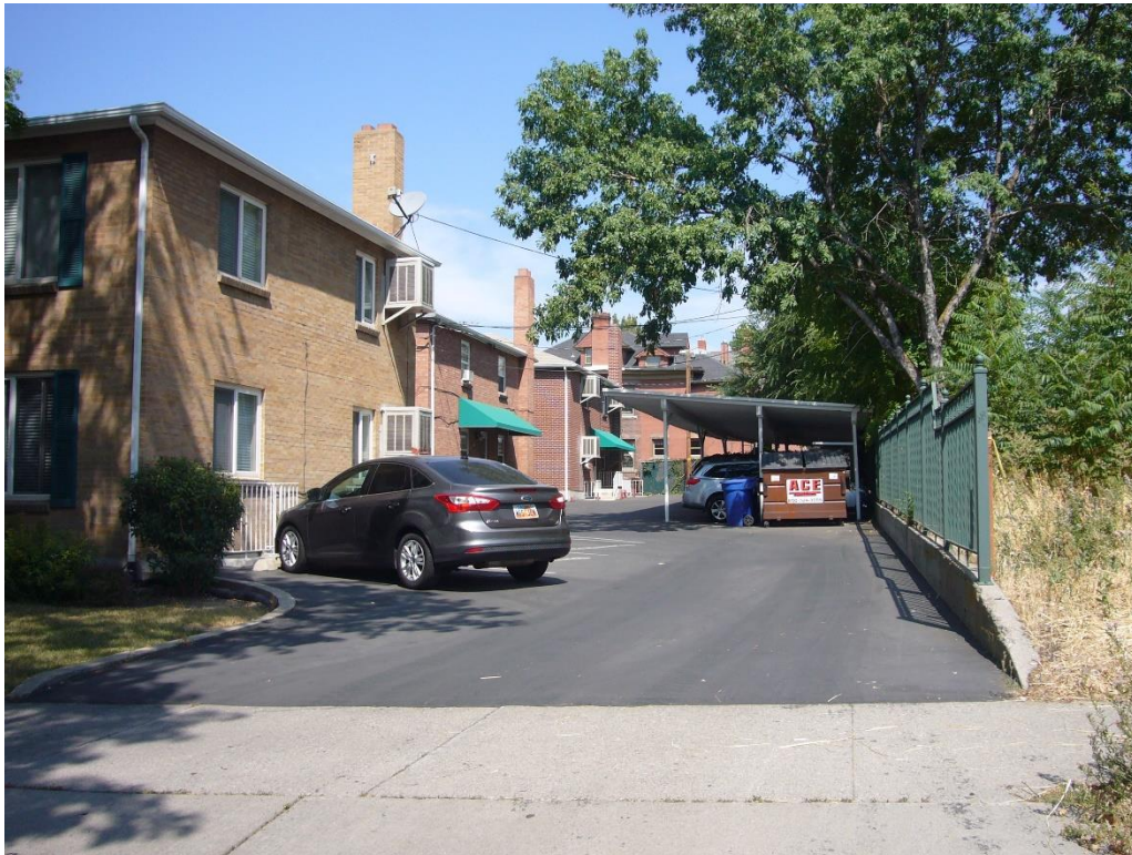
Driveway between the subject property and apartment building to the west
