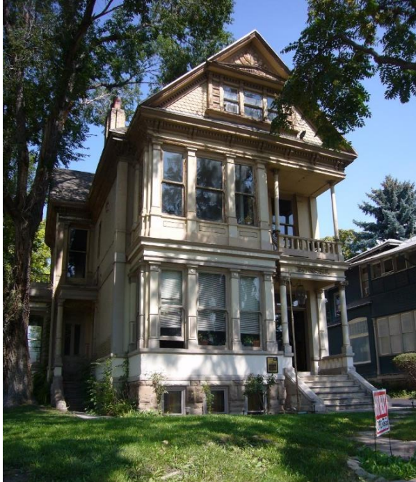
623 East 100 South (Landmark Building)
