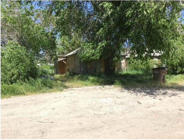
Subject property abandoned structure proposed to be demolished
