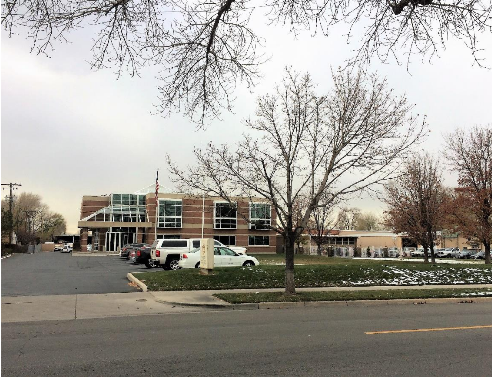
Existing Okland Construction office and frontage along South West Temple.
