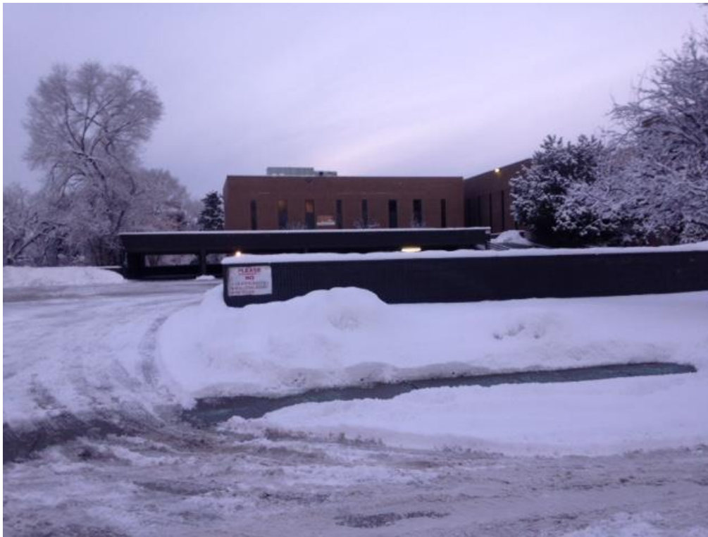
Office building on the north side of the block on 500 South and Denver Street. Wall is approximately 3'5".
