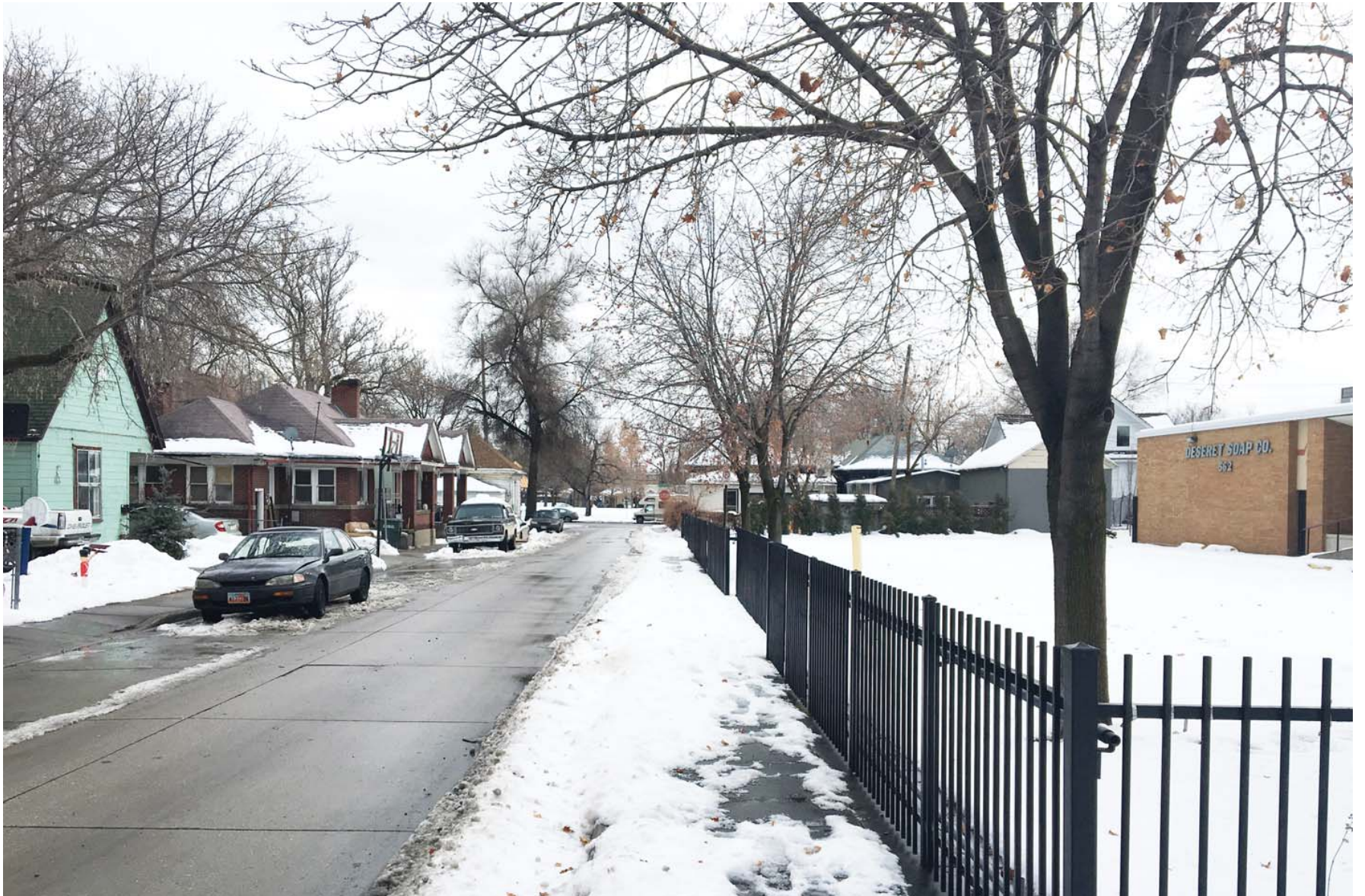
existing 4' high iron fence at sidewalk
