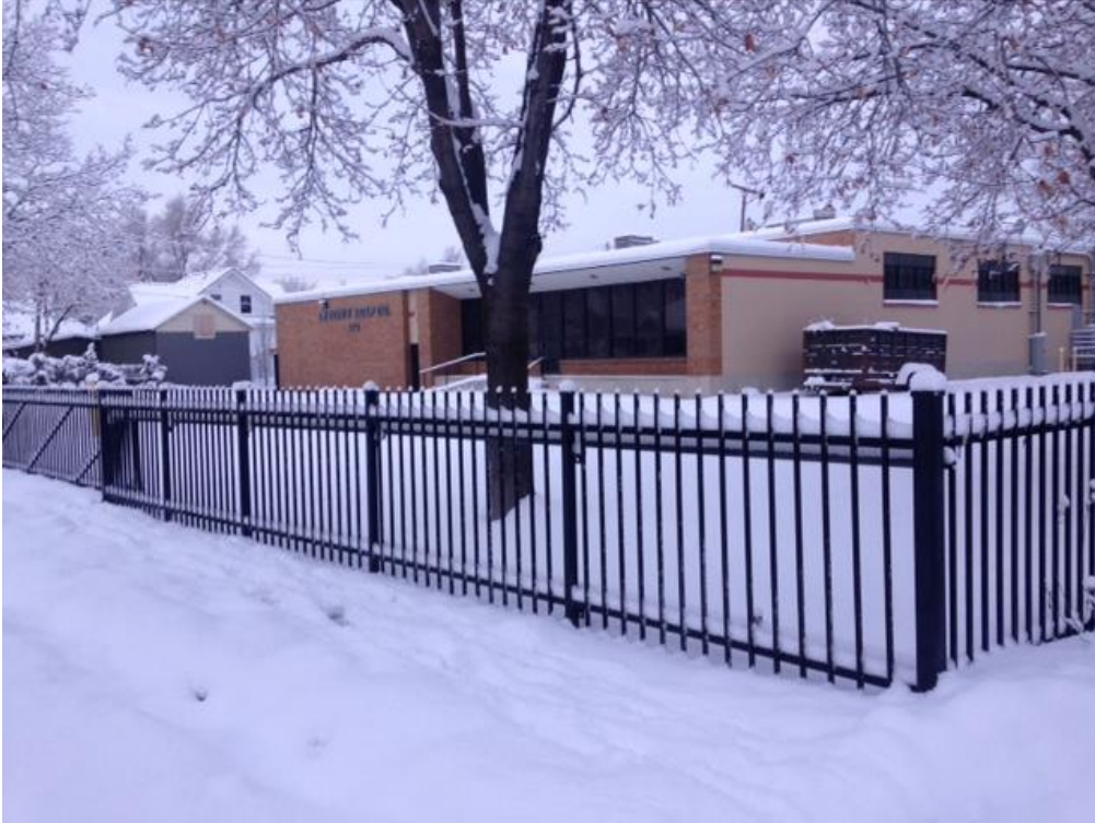
Subject property with existing 4-foot wrought iron fence to be replaced with wall.
