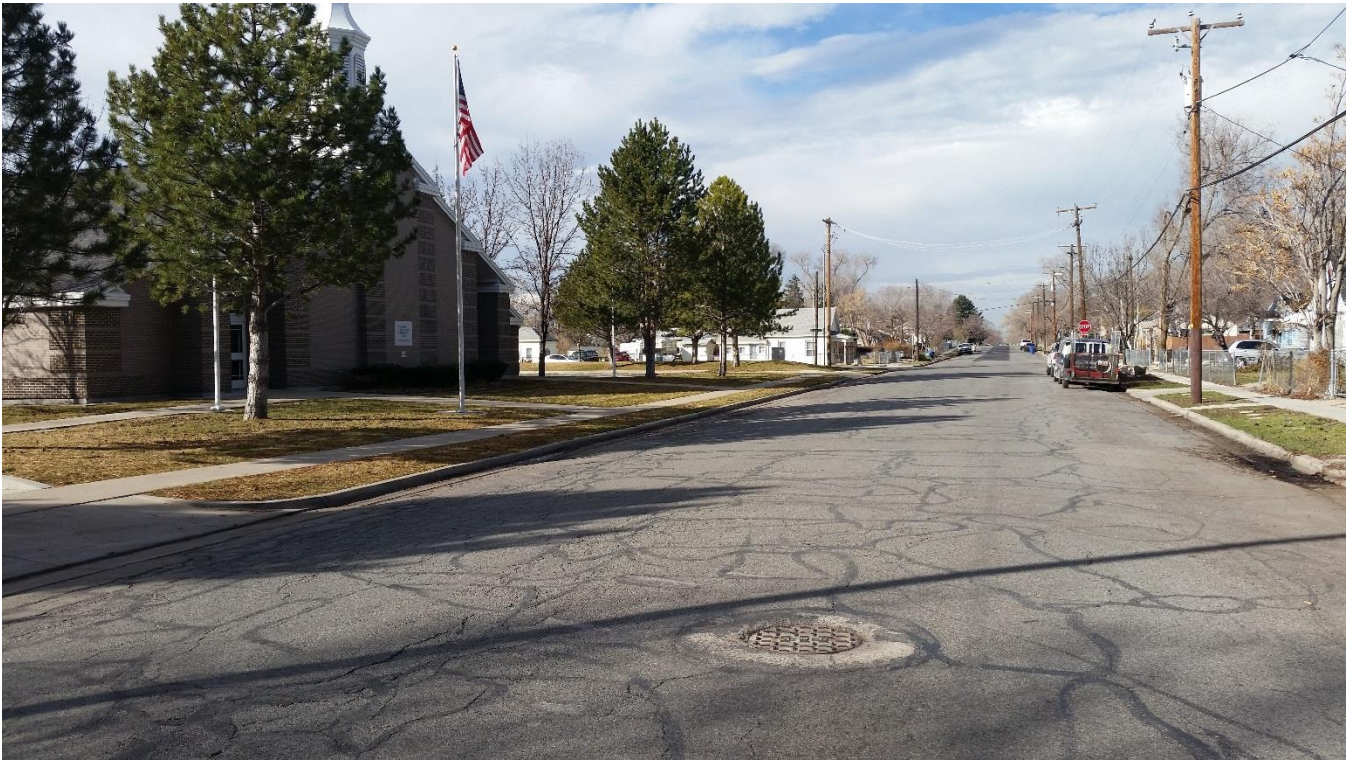
500 South looking southwest
