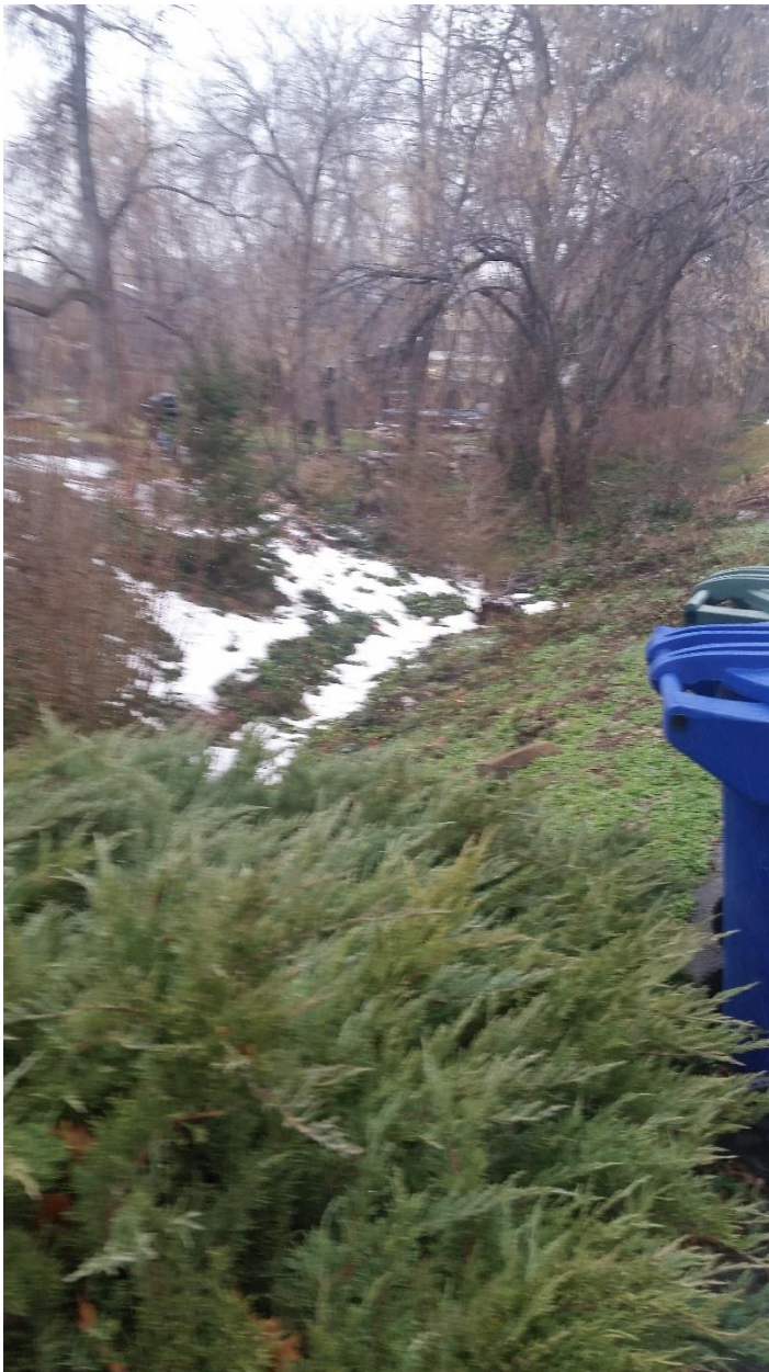
Drainage on south side of lot
