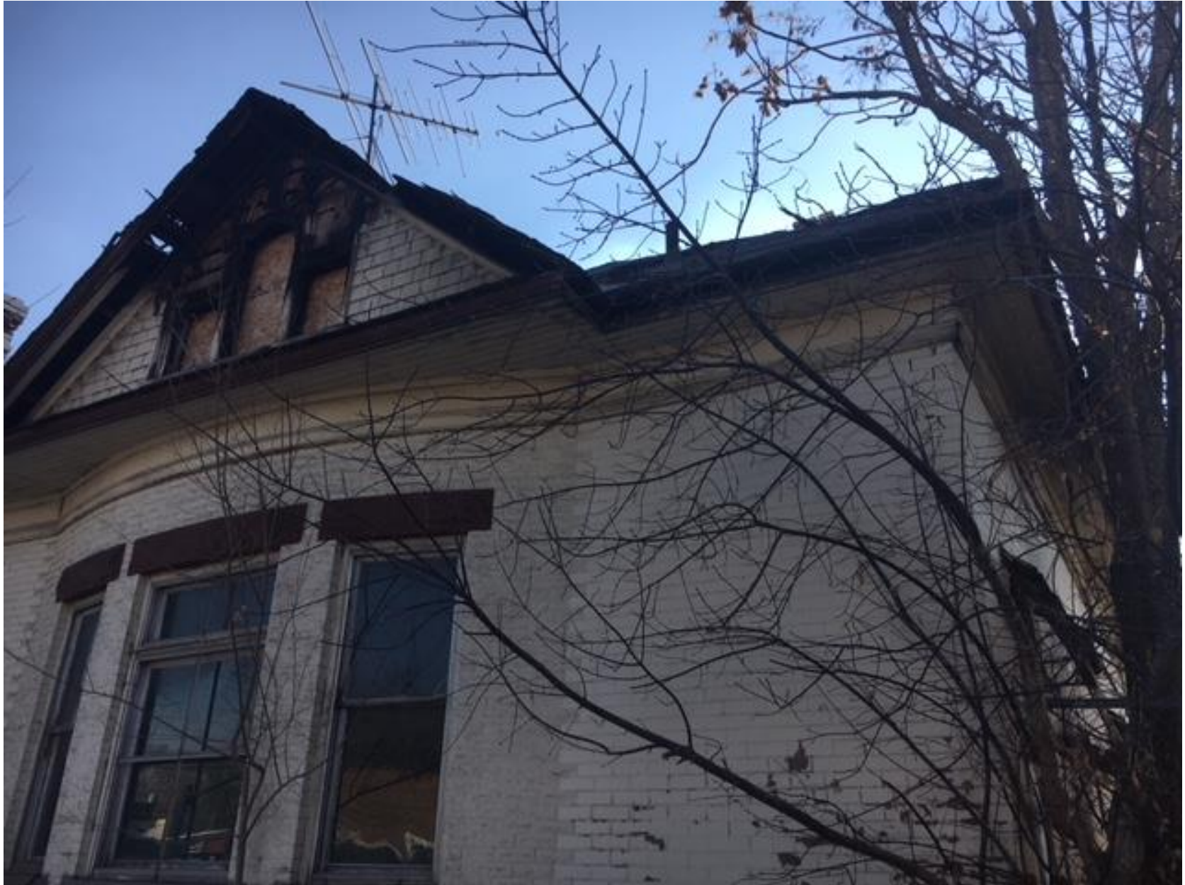
This photograph shows an existing single-family dwelling on the site. It is located on the corner of 1700 S. and West Temple. A fire has left the dwelling uninhabitable.
