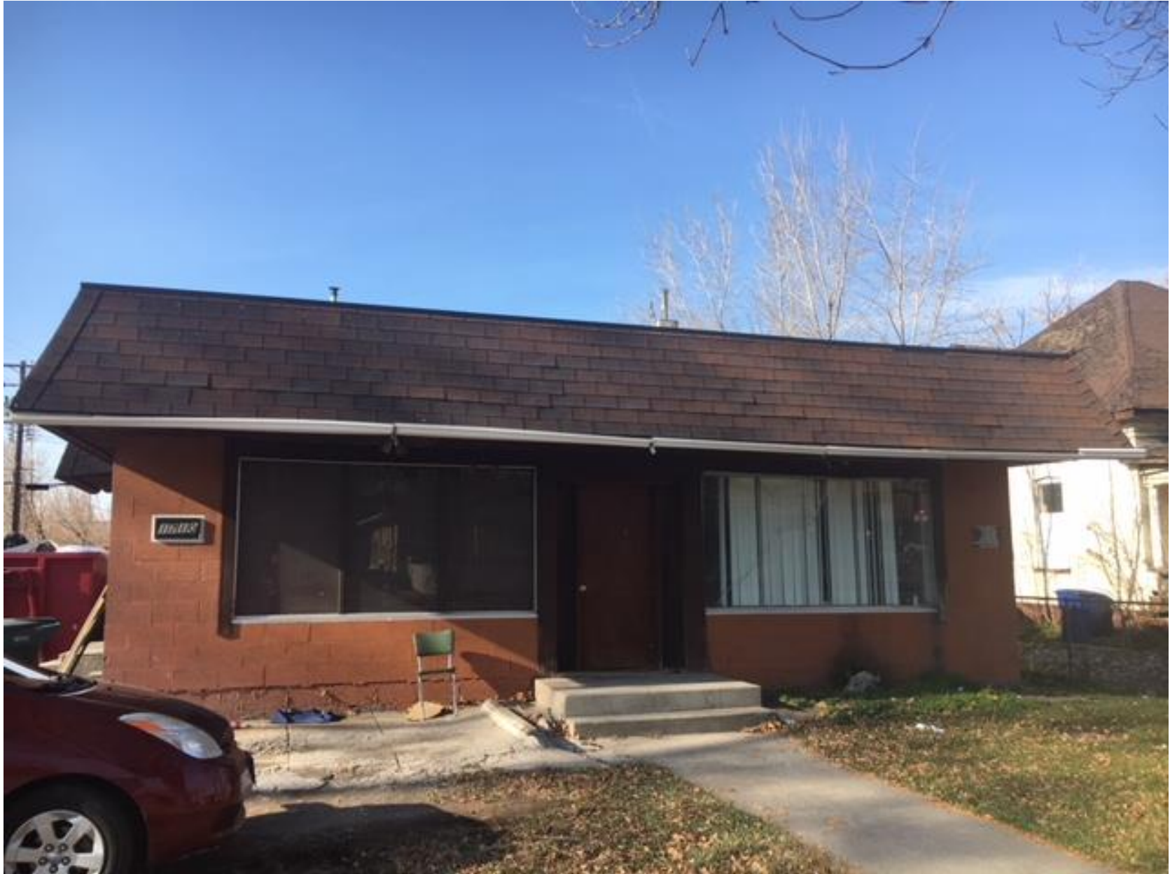
This photograph shows one of the existing commercial structures on the property. This structure is located on West Temple St.
