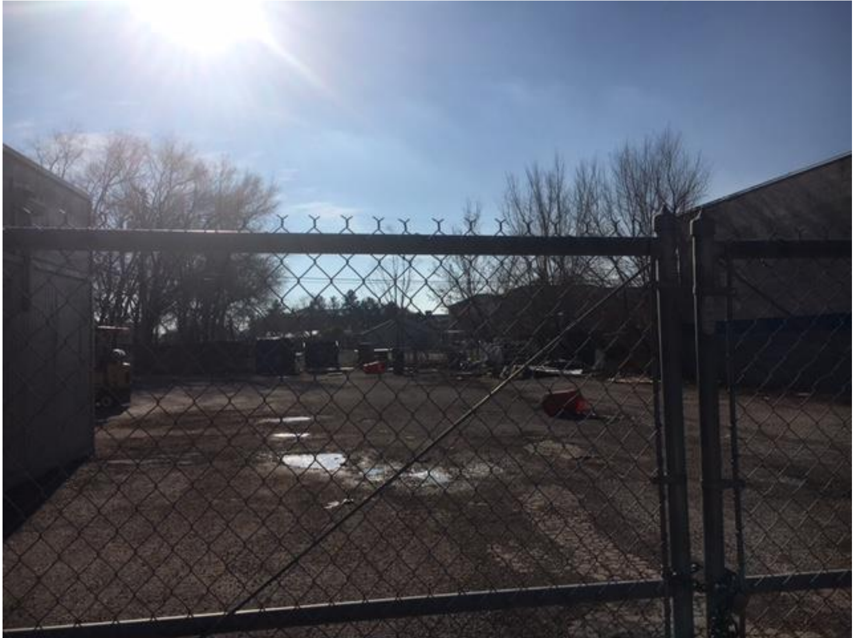
This photograph was taken looking south from 1700 South at the rear yard of the existing commercial site.
