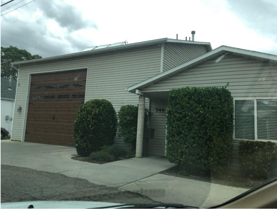
Existing single-family dwelling at 744 W. Jackson Avenue
