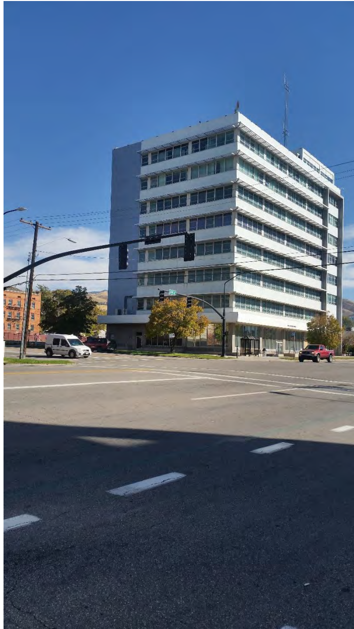
Former Public Safety Building/Northwest Pipeline building to be renovated and preserved.
