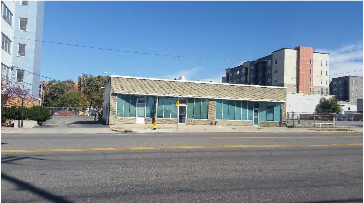
Building to be removed and replaced with plaza and housing
