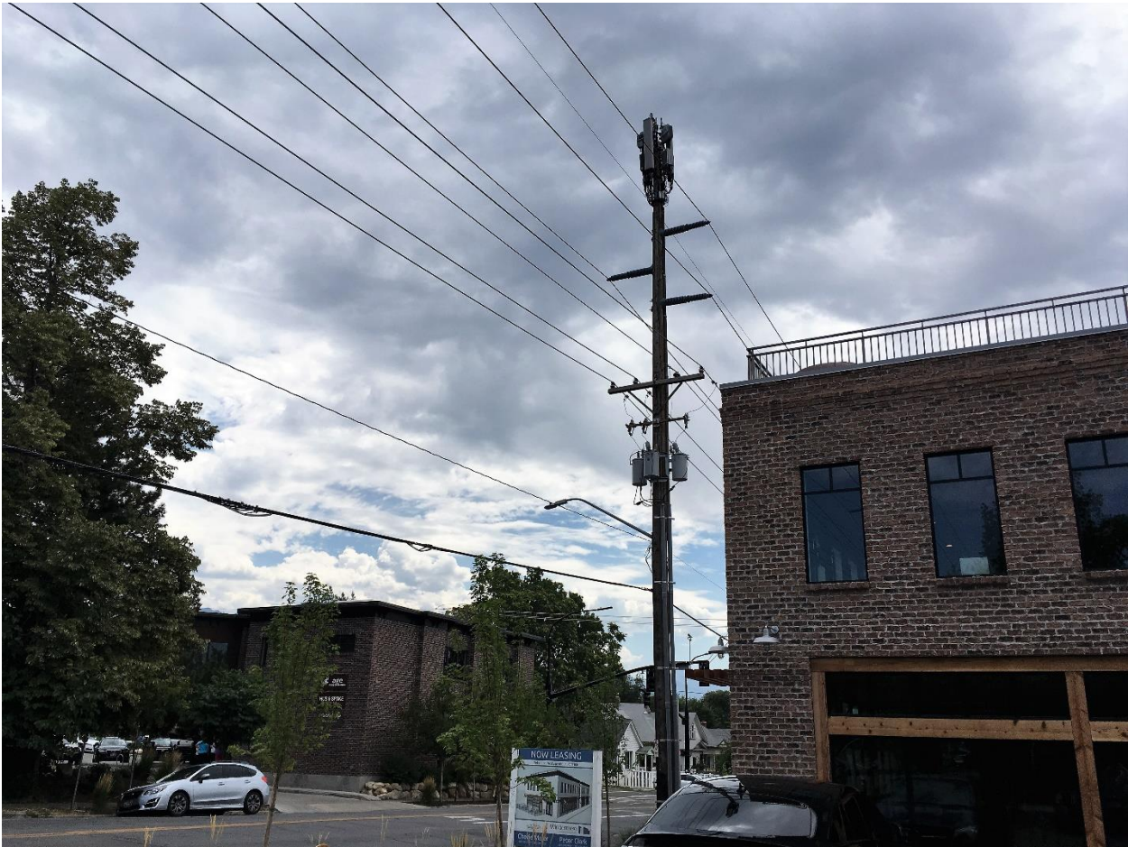
Existing wooden utility pole located in the right-of-way adjacent to a new mix-use commercial building. Pole to be replaced with a steel utility pole and antenna array to be expanded.
