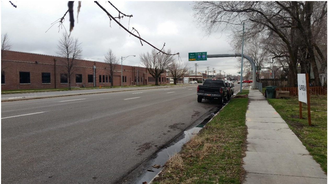
West Temple and data center (former soft drink manufacturing site) across the street
