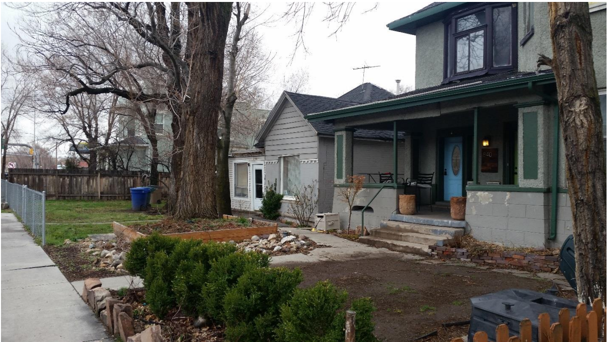
Homes to the south of the site (to remain)
