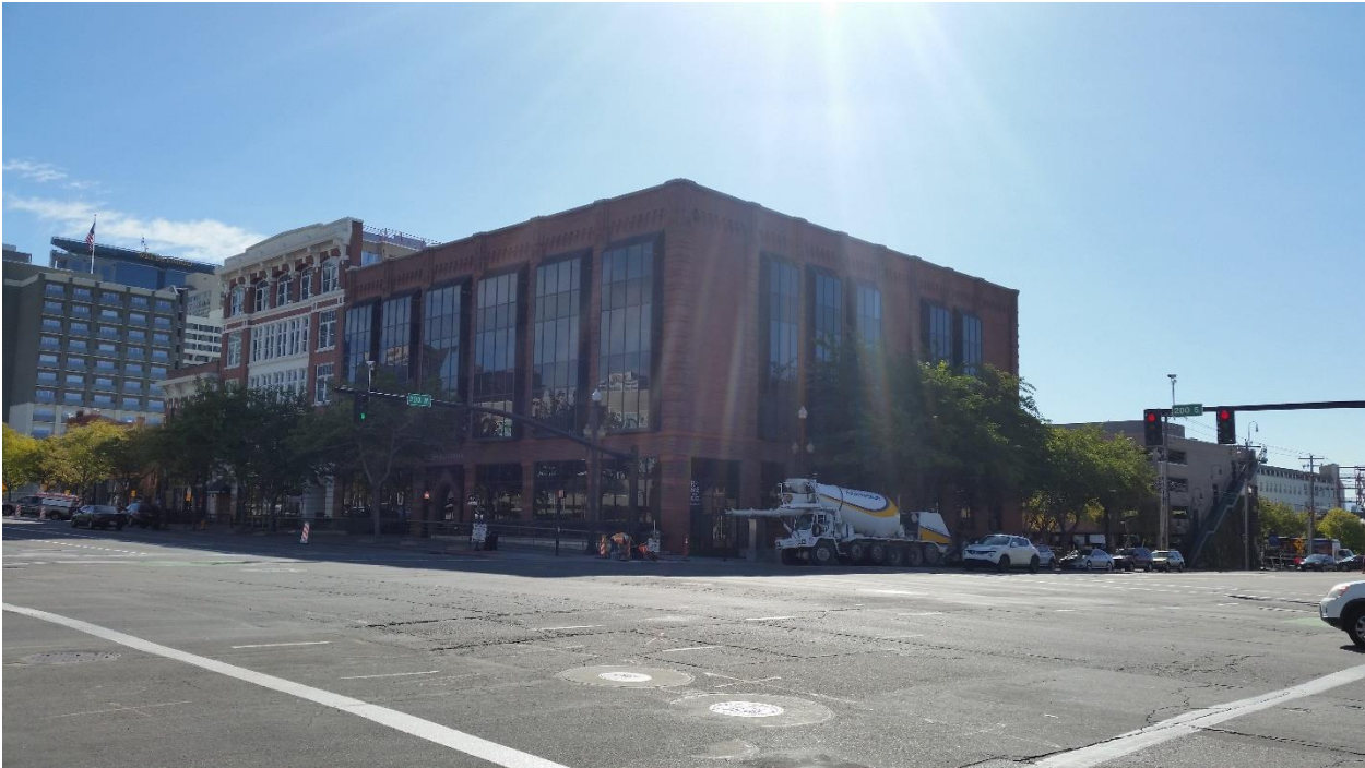
Office building to southeast
