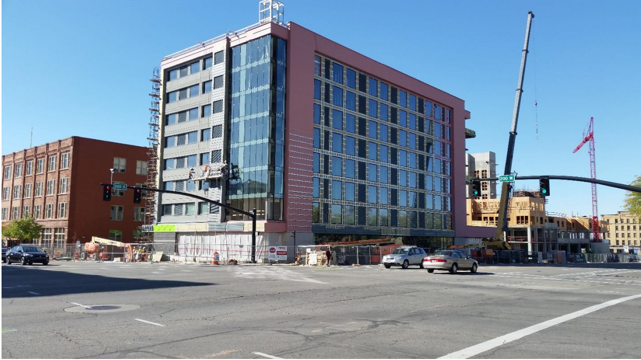
New hotel and apartments being constructed to the south
