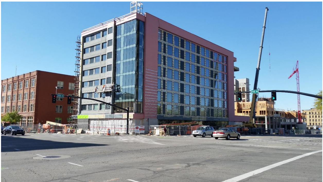
New hotel and apartments being constructed to the south
