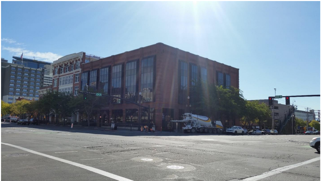
Office building to southeast
