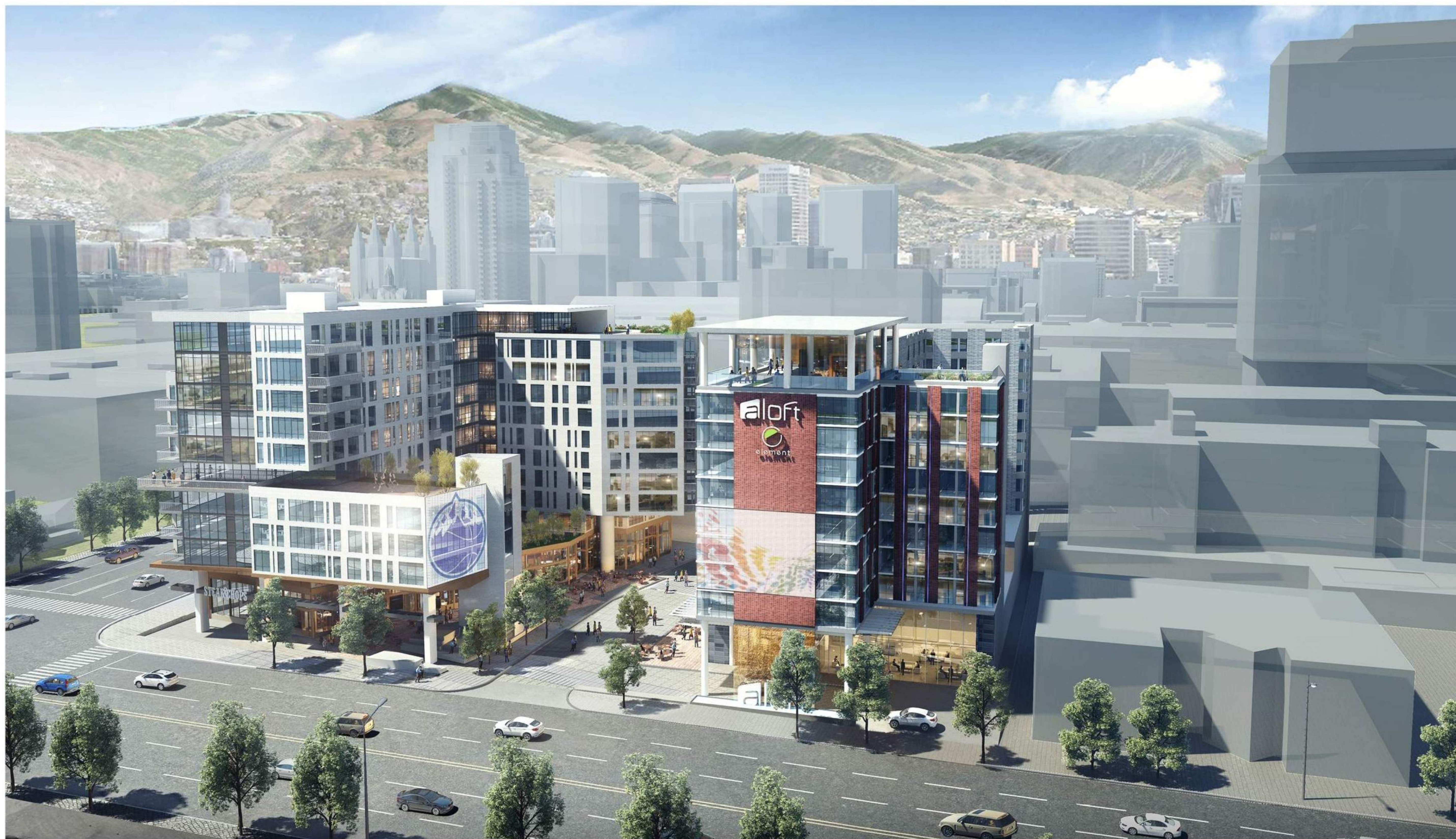
Aerial view looking Northeast towards downtown
