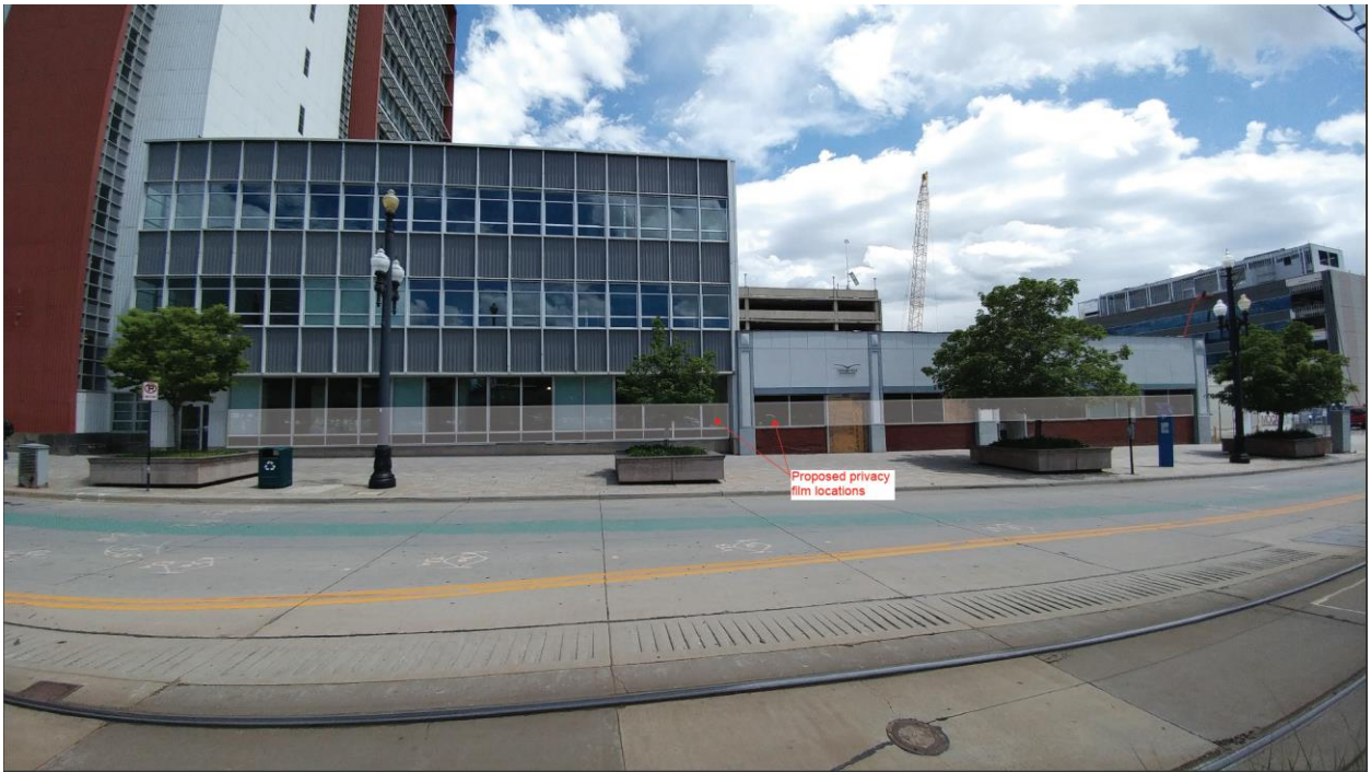
The image above displays the windows that are proposed to be covered.
