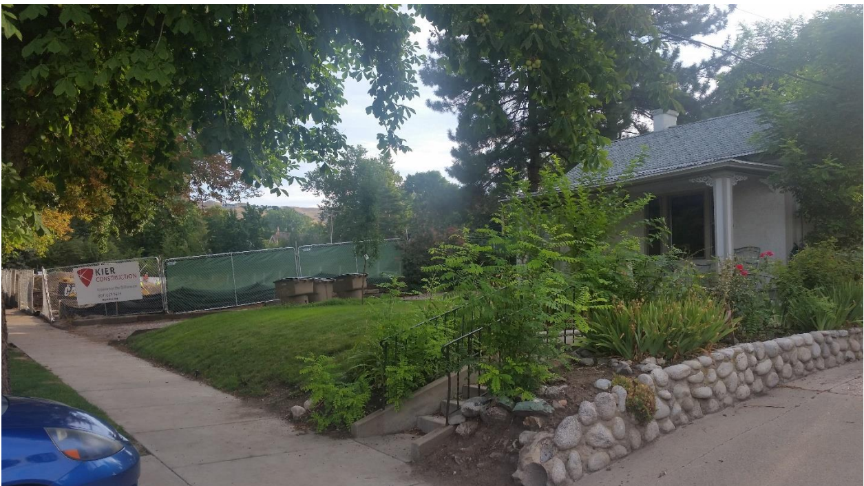
900 East looking northeast (the home in the photo is directly north of the boarding house, the construction in the photo is for a new apartment building)
