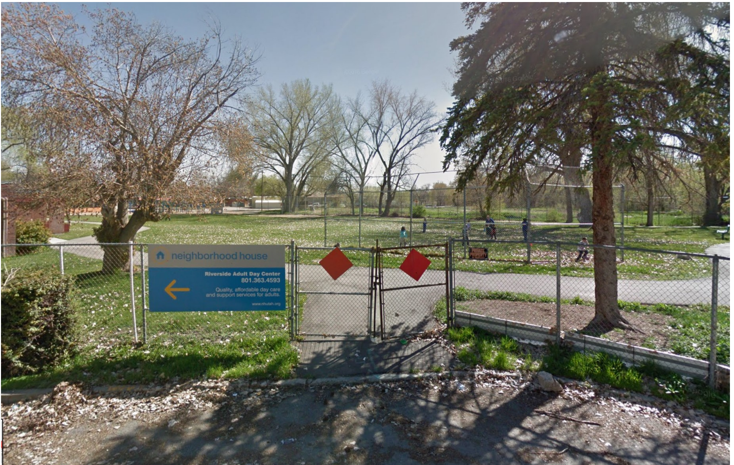
View of the portion of the street to be closed, beyond the gate.
