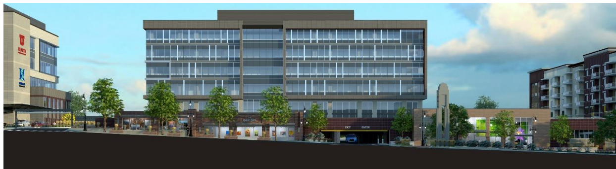
View of the parking structure (ground level) and Office B
