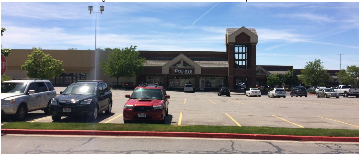
View looking west toward existing Shopko building (to be torn down) and Payless retail space (to remain) within the Sugar House Shopping Center building. The property line runs along the shared building wall.
