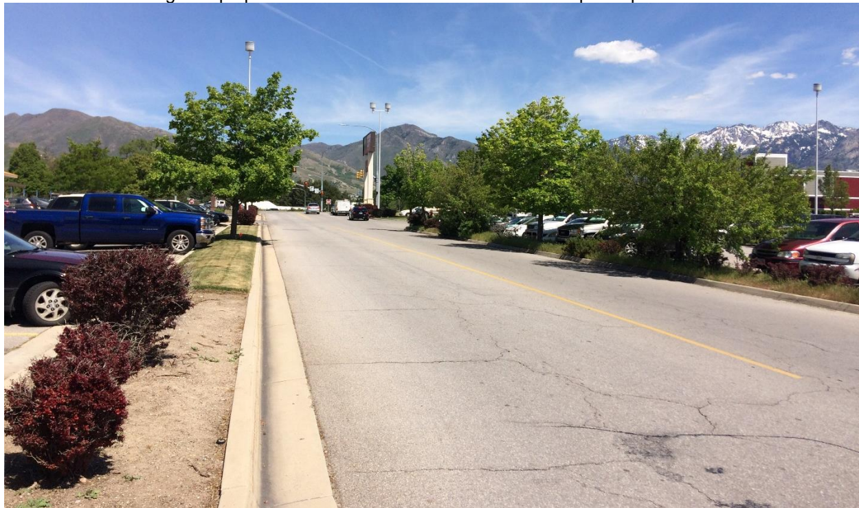
View looking east of current configuration of the drive that will be reconstructed as a street with pedestrian sidewalks and amenities
