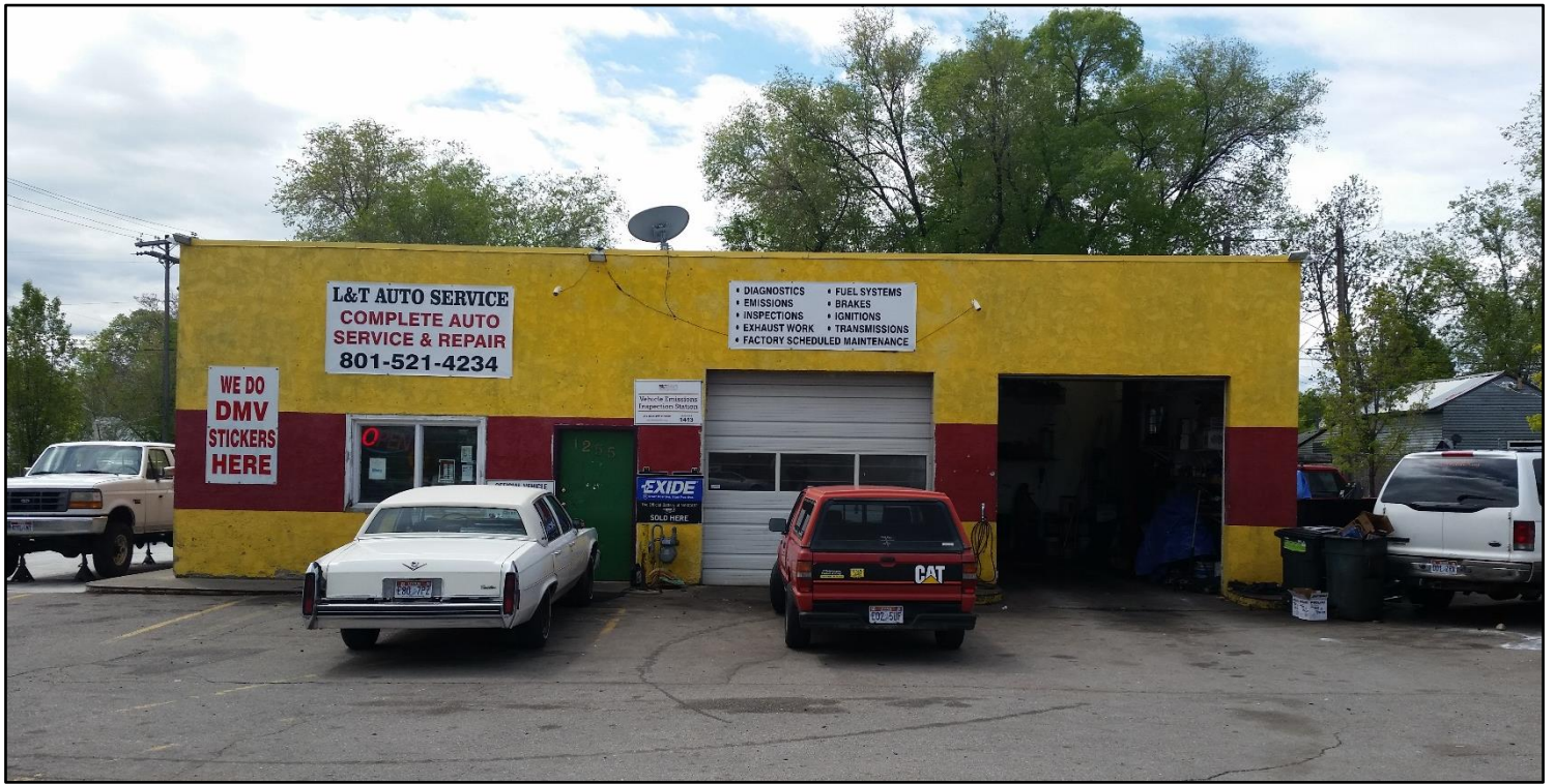
View of the entrance and two existing bays on the north side of the building
