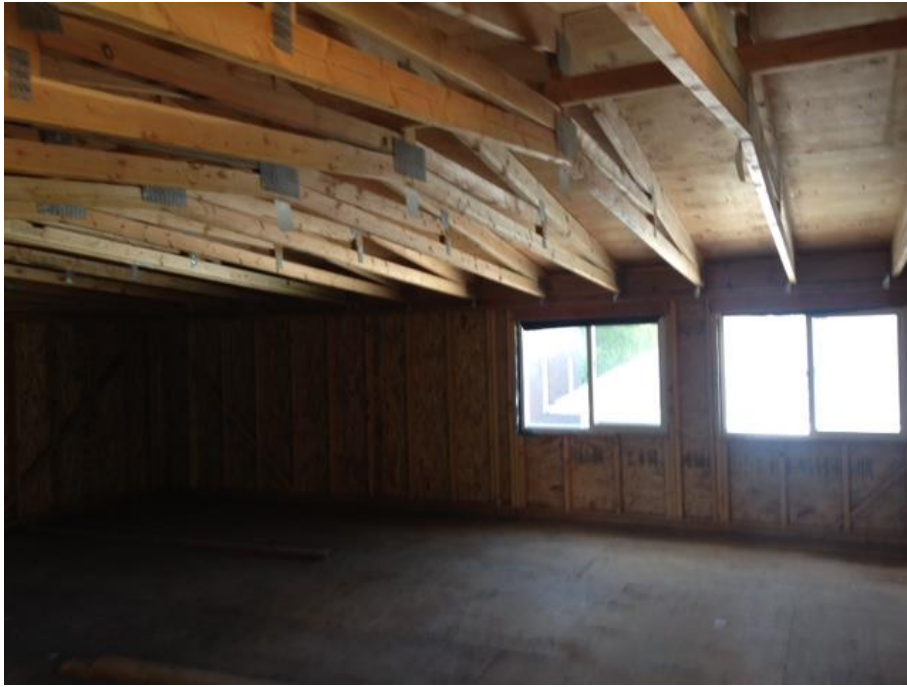
Inside the second story of the garage facing south where proposed hobby shop will be located.
