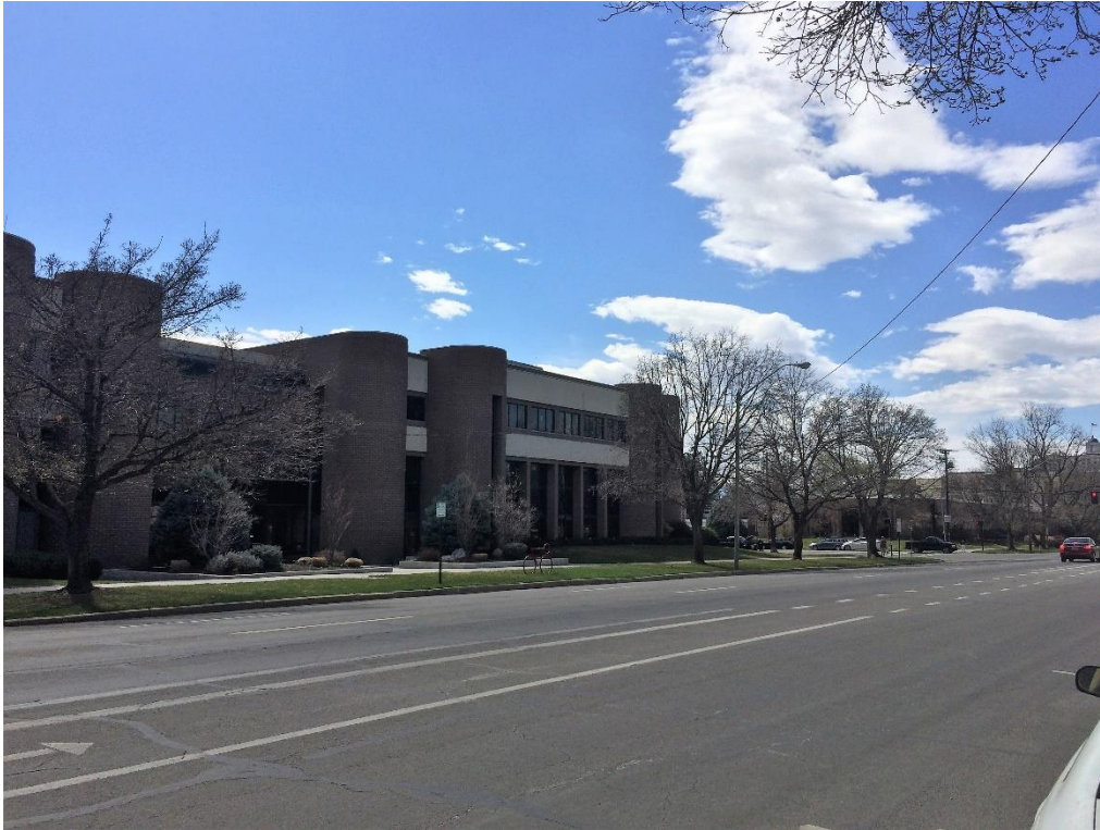
View looking southeast across 500 S at the subject property.
