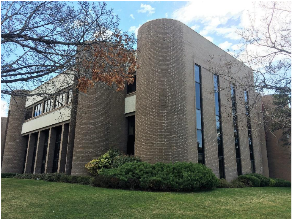
Northeast property corner at 500 S 400 E showing existing buildings.
