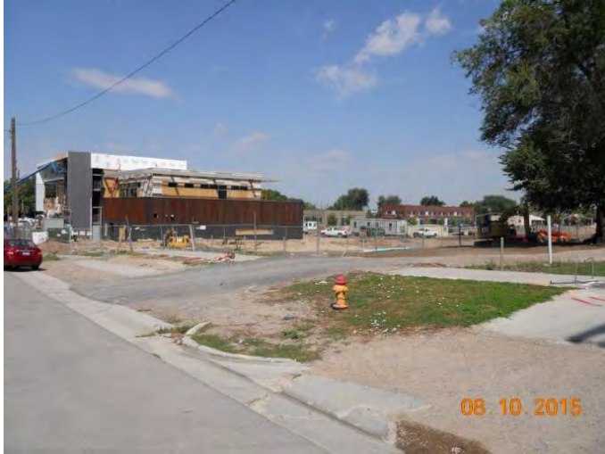
View of project site between Arctic Court and the proposed park plaza and the Marmalade Library from 500 North looking north. The project site is located between Arctic Court and the chain link fence shown in the photo
