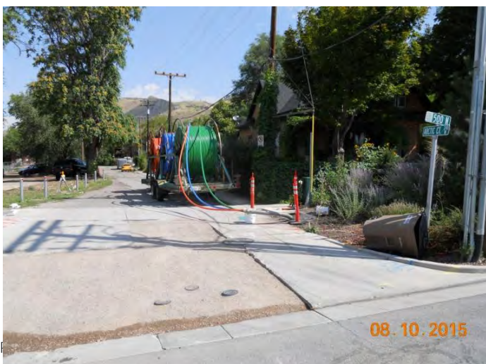
View of Arctic Court from 500 North looking north.
