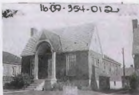
1392 E. Laird Ave Built : 1927 Neoclassical/English cottage
