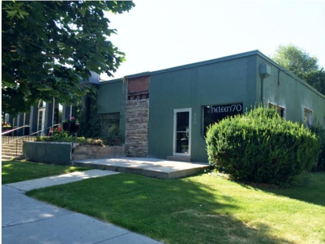
Front (North) View
