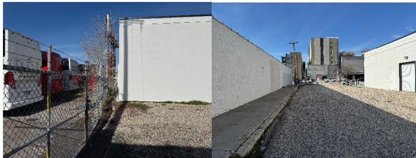
(Above Left) West side North facing. (Above Right) West side East facing.
