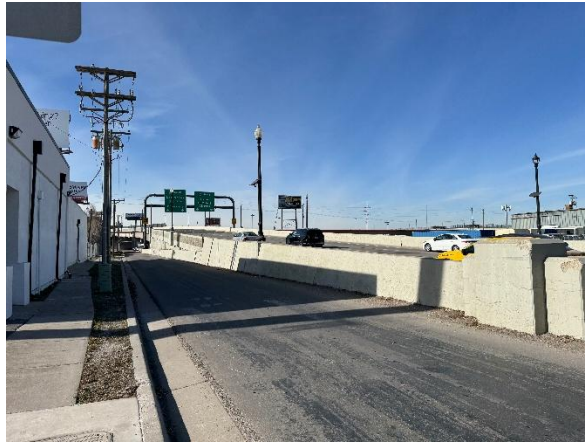
(Above) North side of the property is 500S freeway entrance West facing
