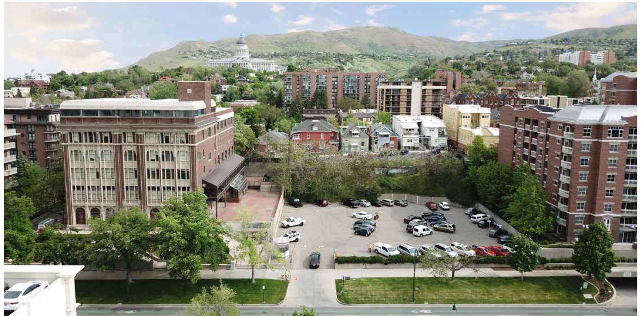
Existing Site Condition
