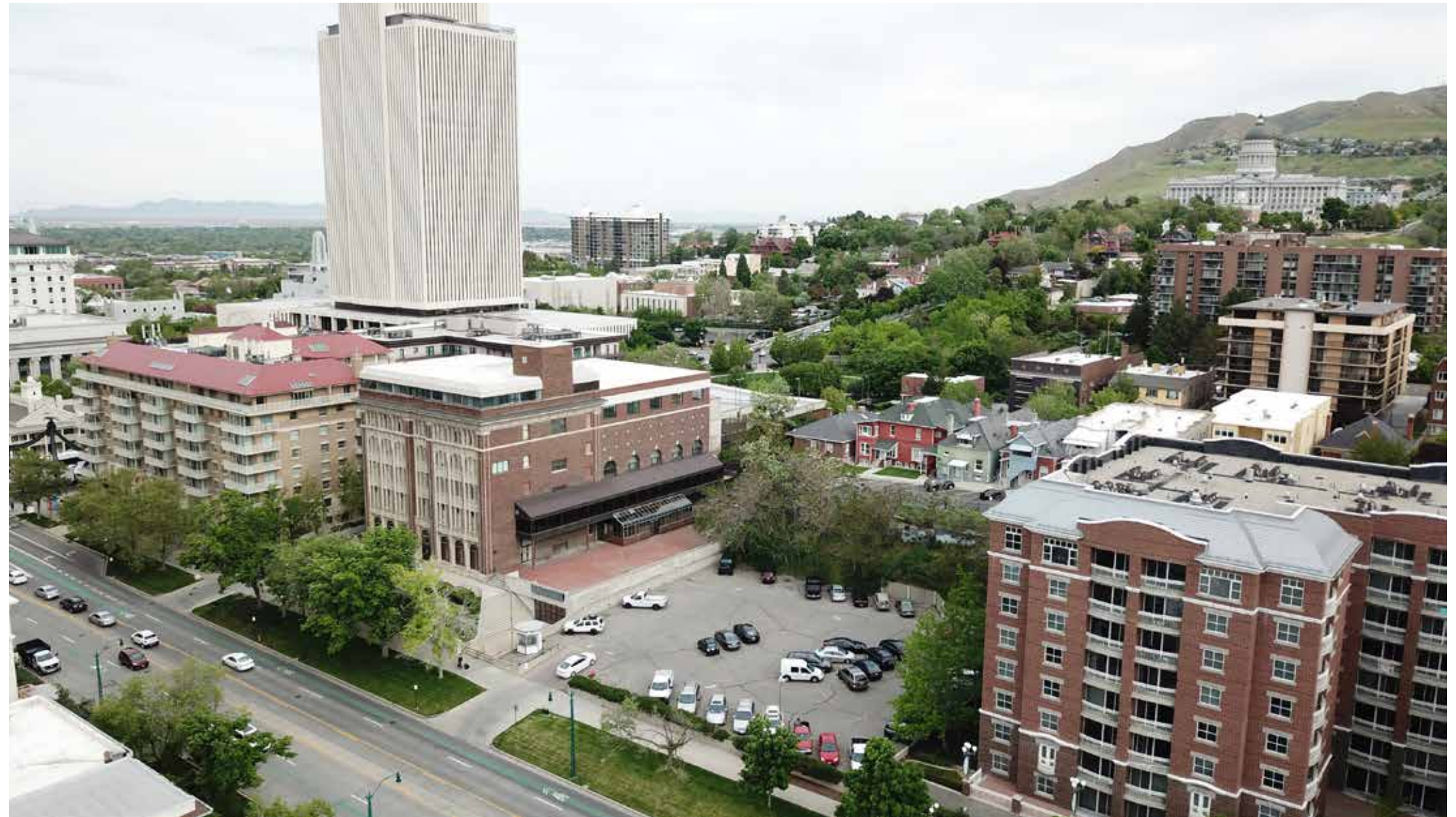
Existing Site Conditions in 2020
