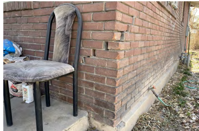
Home 5— Detail view of structural issues, foundation bowing outward.
