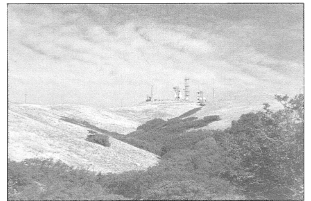
Communications tower corridor in the foothills
