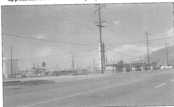
Major industrial uses
