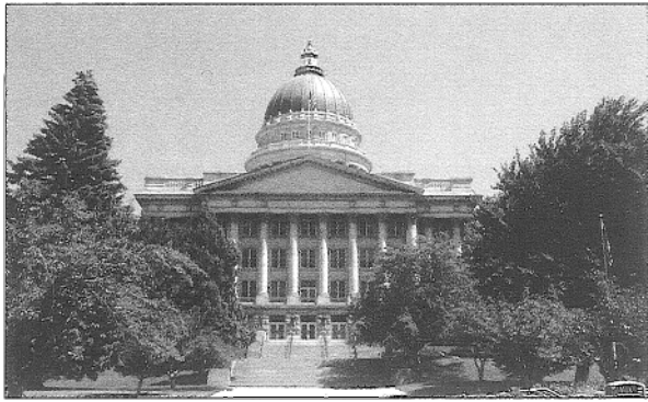
Utah State Capitol Building
