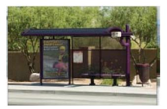
Solar roof systems are integrated with kiosks and benches to create a transit shelter
