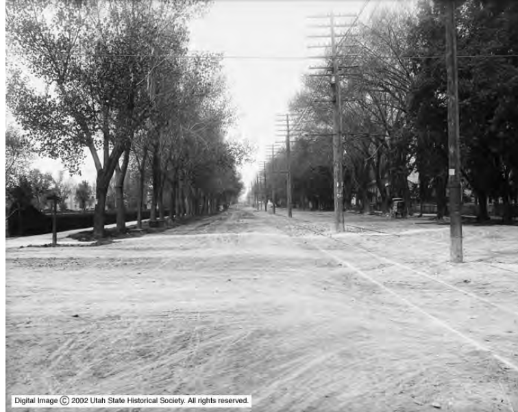
Figure 4.1.3: 1909 photo of street paving looking south along 400 West. Pioneer Park is visible on the left-hand side of the historic image. This photo illustrates the sidewalk, park strip and street tree configuration defining the perimeter of the park. A clipped hedge lined the inside of the public sidewalks. A portion of the corner entrance to the park is visible.
