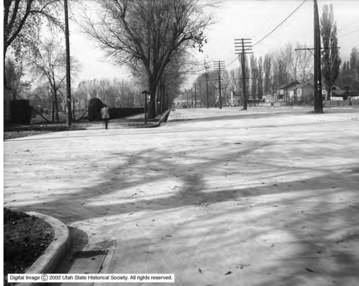
Figure 4.1.1: 1909 photo of street paving looking west along 300 South. Pioneer Park is visible on the left-hand side of the historic image. This photo illustrates the sidewalk, park strip and street tree configuration defining the perimeter of the park. A clipped hedge lined the inside of the public sidewalks. The corner entrance to the park is visible.
