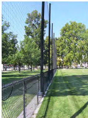
S14. Fence with Light Poles
