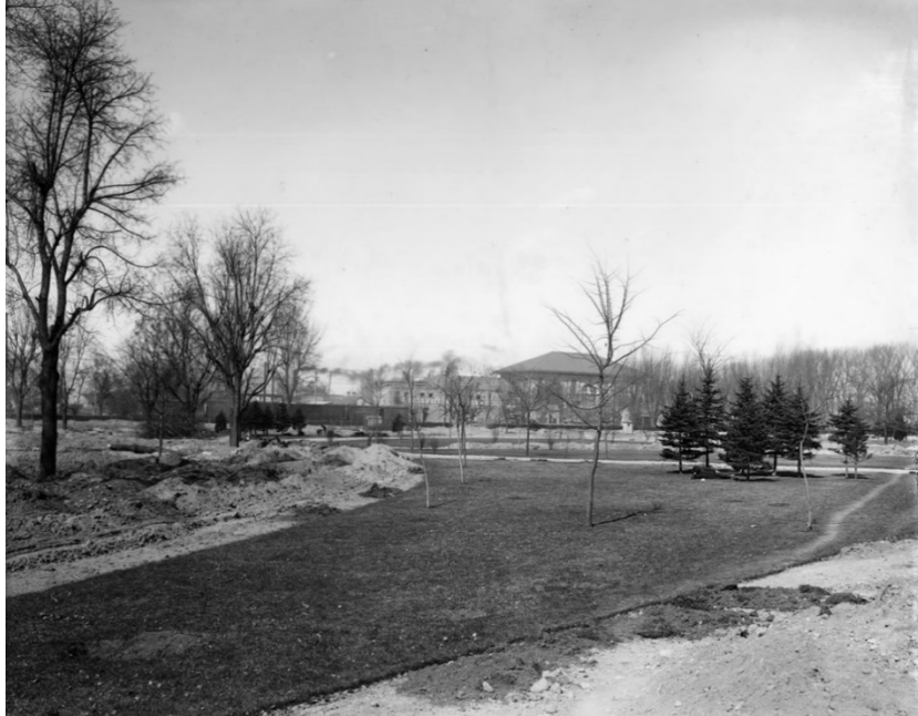
Figure 4.2.1: Late 1910 photo looking northwest across the park, with the Denver & Rio Grande Depot visible in the background. The piles of dirt visible in the foreground and on the left indicate that this image was taken mid-construction.
