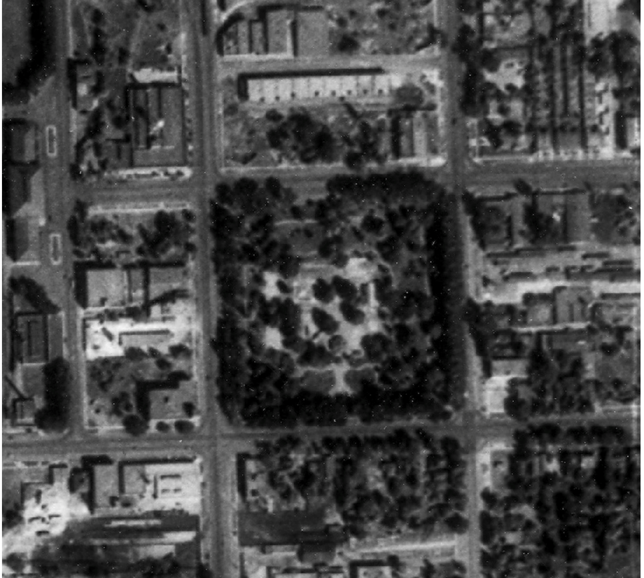
Figure 4.12.1: 1937 aerial photo. This image illustrates the dense tree canopy that was beginning to mature toward the later end of the Americanization Period. Openings in the canopy reveal the regimented ground-plane with Beaux Arts geometry, including symmetry in the entry sequence to the park extending north from 400 South. Mid-block cardinal and diagonal pathways are visible in this image, along with two interior perimeter pathways. The tennis courts, pools, and some of the buildings are also visible.
