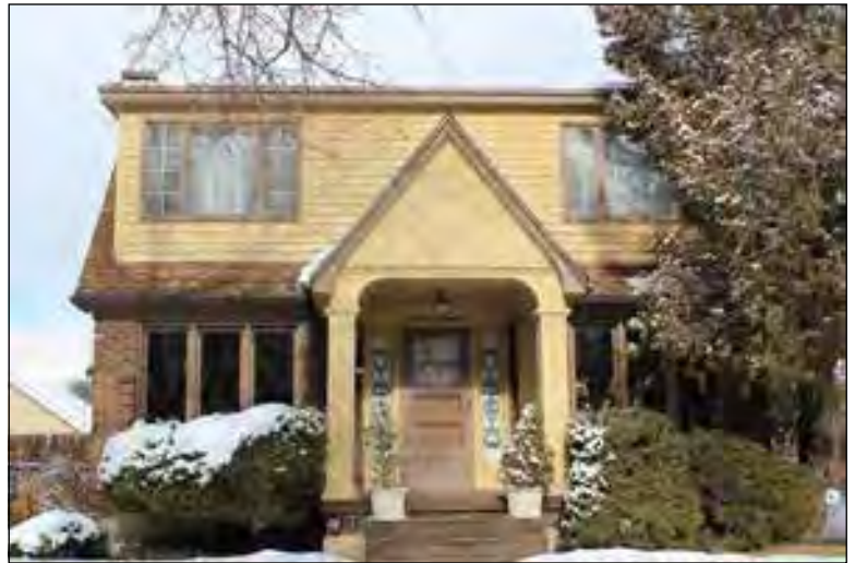
1719 Yale Ave. Built c. 1926 Striated brick with half timbering Neoclassical/Period Revival:Other
