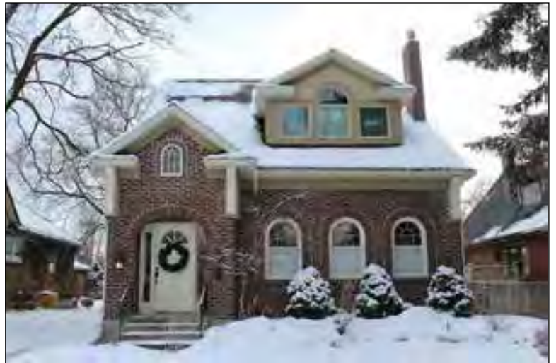
1714 Yale Ave. Built 1926 by P. Biesinger Aluminum/vinyl siding with striated brick English Cottage, other unclear style
