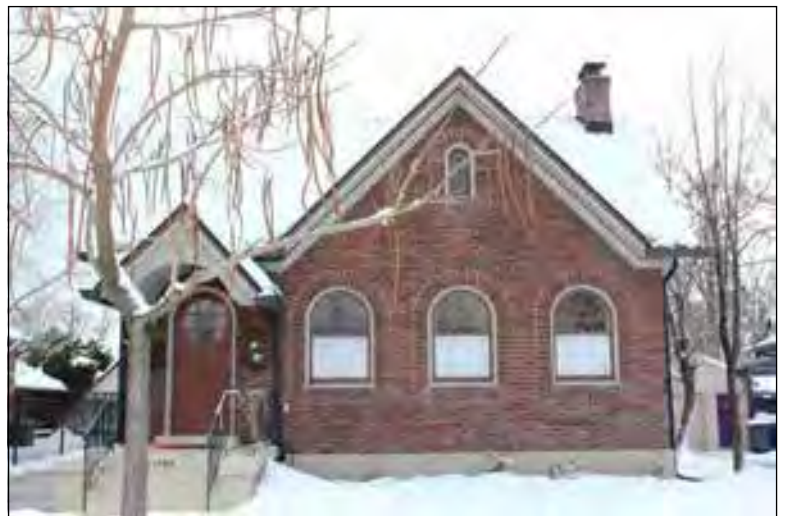
1762 Yale Ave. Built 1926 by H. Biesinger Regular brick with half timbering English Cottage
