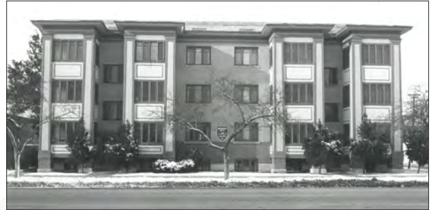
Browning Apartments, c. 1916, Ogden, Weber County. Constructed for Ogden businessman George E. Browning, this horizontal block shows the influence of the prairie School style in the use of casement windows and wood banding.
