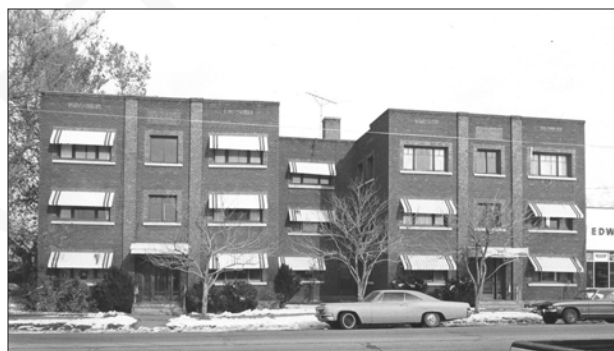
Rose Apartments, 1923-24, Ogden, Weber County. This is a brick masonry “C”-shaped apartment building containing entries in the wings.
