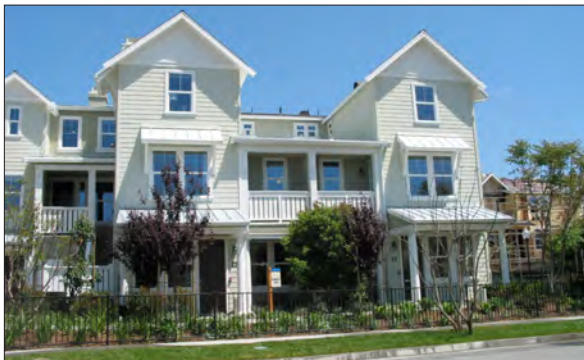
Gabled full height wings frame recessed floors and balcony space creating a strong sense of human scale and visual interest.
