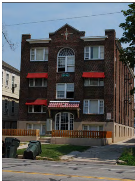
Central approach, entrance and axial 'pedimented' bay help to enhance the coherent, symmetrical contribution to the street.
