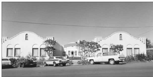
Apartment court, c. 1920, Price, Carbon County. A one-story “U” court of stuccoed masonry, this apartment building shows the influence of the Mission style.
