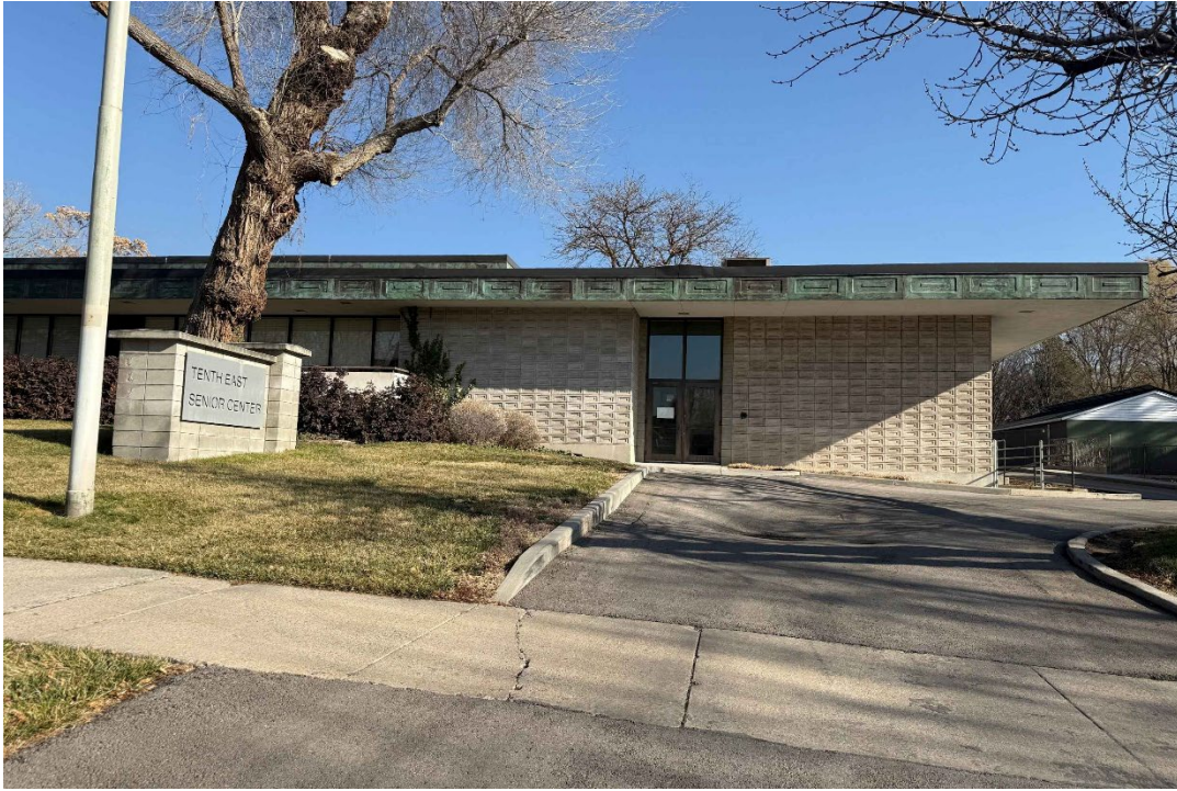
Photograph 5 West elevation including the 1983 addition (right). Camera facing east.
