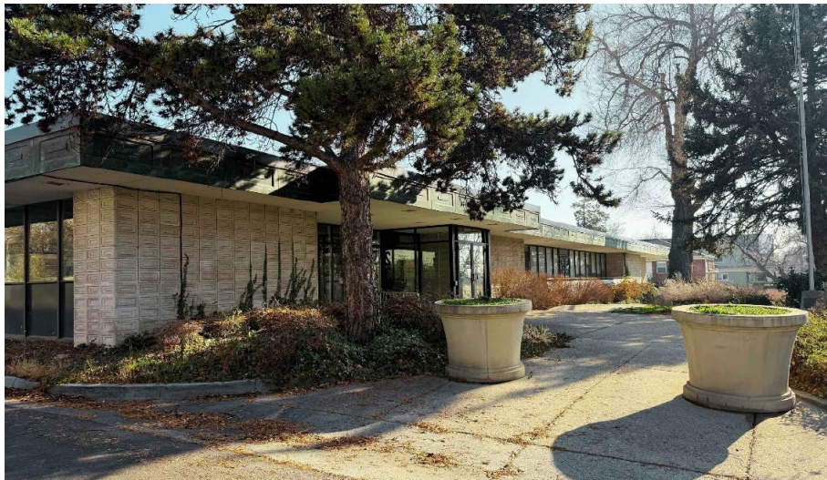
NORTHWEST ELEVATION -LOOKING SOUTHEAST FROM 1000 EAST
