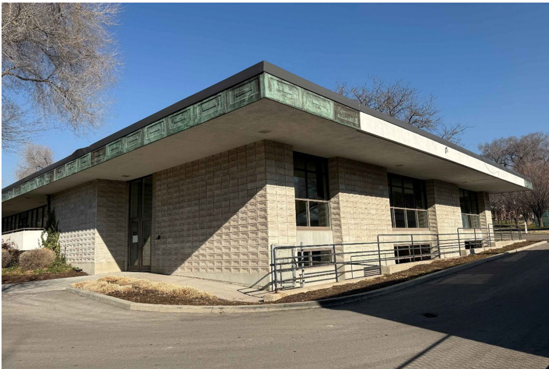
Photograph 6 West and south elevations including the 1983 addition (right). Camera facing northeast.
