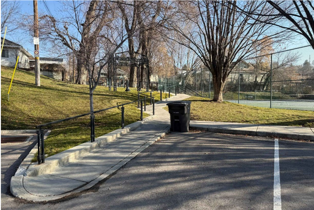
Photograph 21 Western entrance to Victory Recreation Park. Camera facing southeast.
