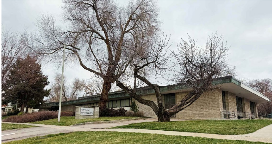
WEST ELEVATION – LOOKING NORTHEAST FROM 1000 EAST
