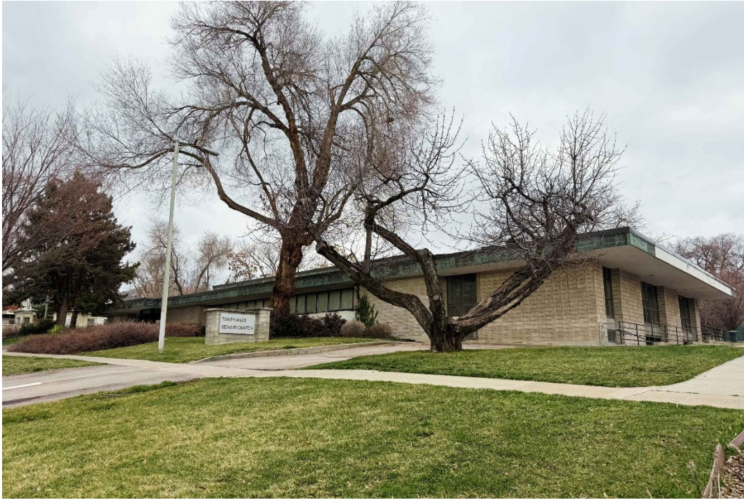
Photograph 1 West elevation of the Tenth East Senior Center. Camera facing northeast.
