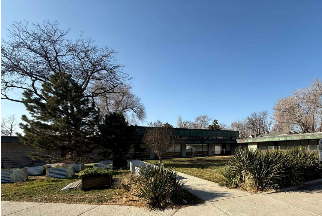
Photograph 15 The Tenth East Senior Center's eastern courtyard. Camera facing northwest.
